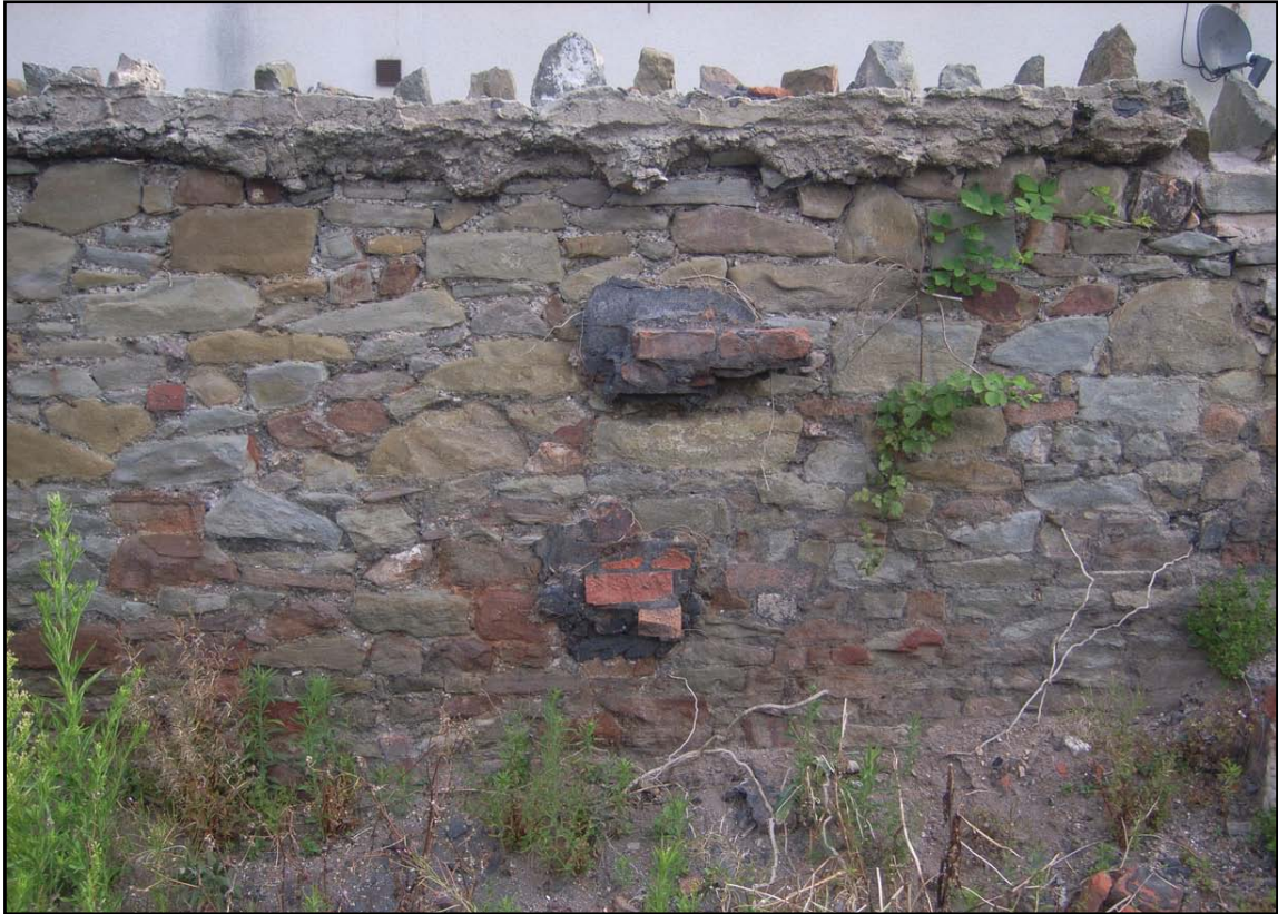
Plate 4 Black 19th-century mortar adhering to the north boundary wall, from the south
