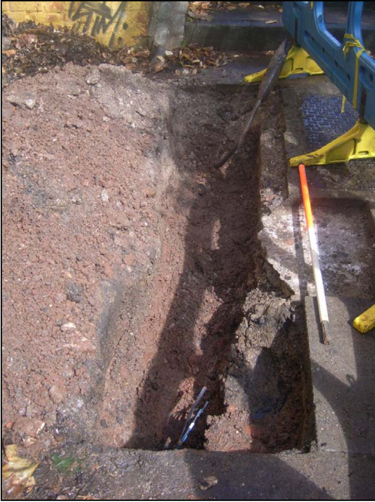
Plate 1 The cable trench after excavation, from the south
