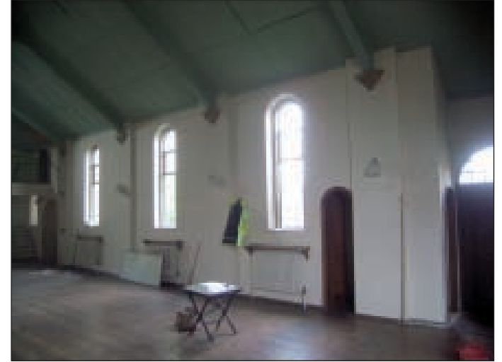
Plate 15 North wall of nave, looking north-west
