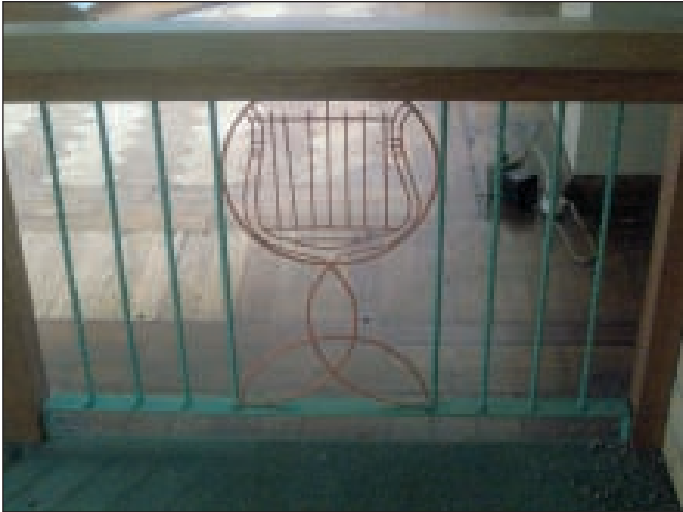
Plate 26 Communion rail ironwork - chancel arch, south end
