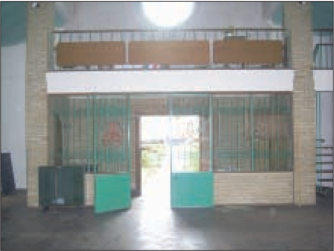
Plate 11 West gallery and narthex beneath, from east
