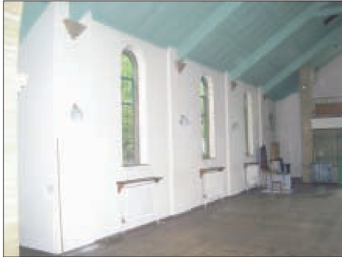
Plate 14 South wall of nave, looking south-west
