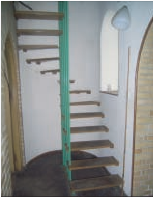
Plate 10 Gallery staircase, looking west
