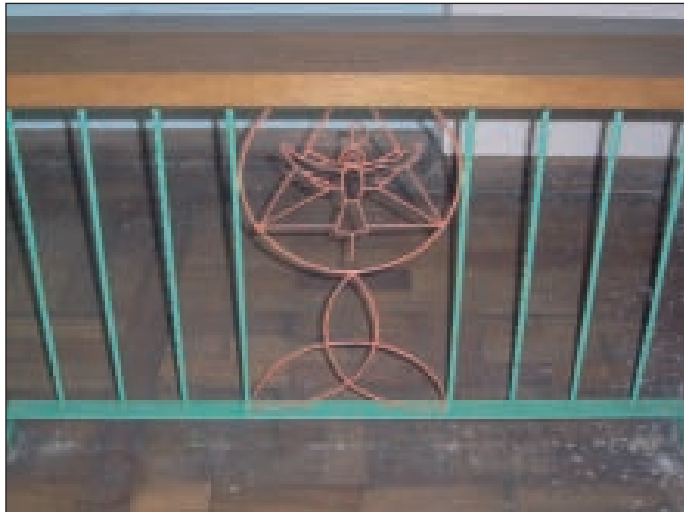
Plate 28 Communion rail ironwork, southern arch, south end
