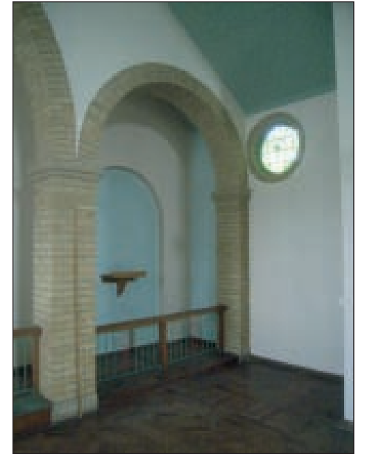
Plate 18 South transept and side chapel, from north-east
