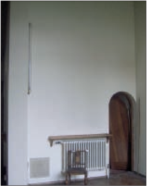
Plate 30 Chancel north wall, looking north-east
