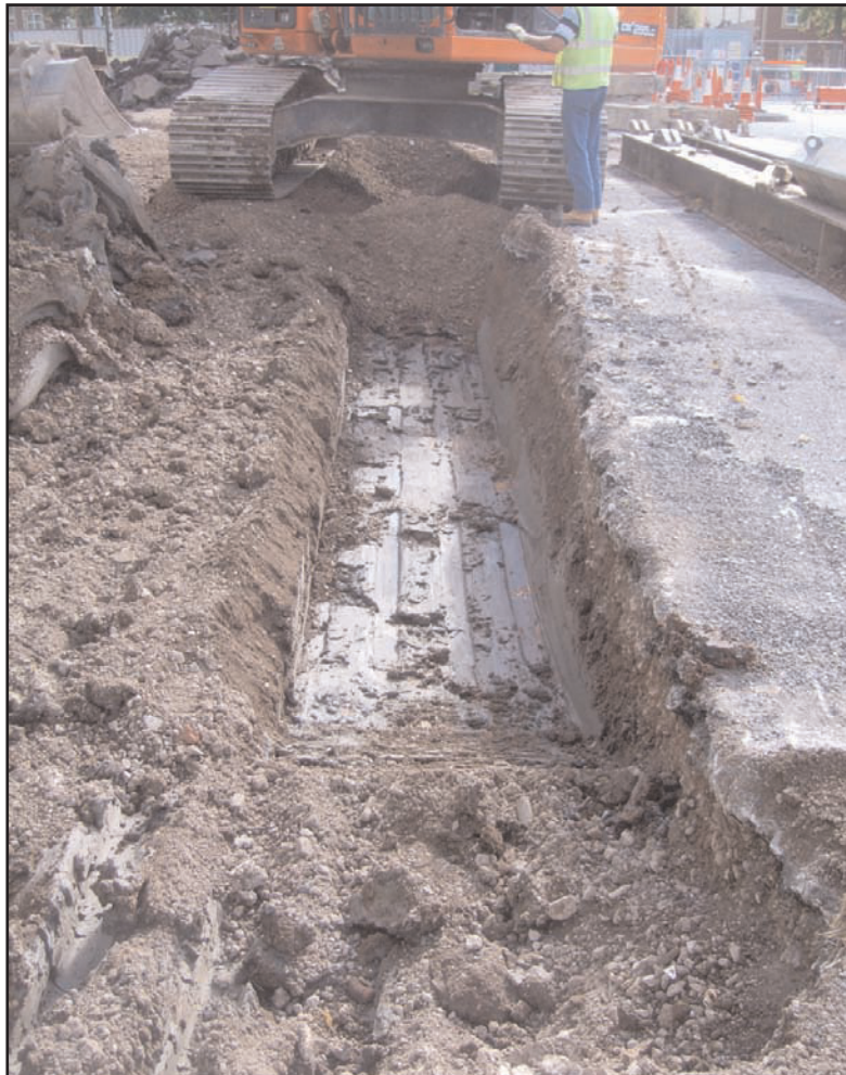
Plate 1 Looking east at the large fuel tanks during excavation
