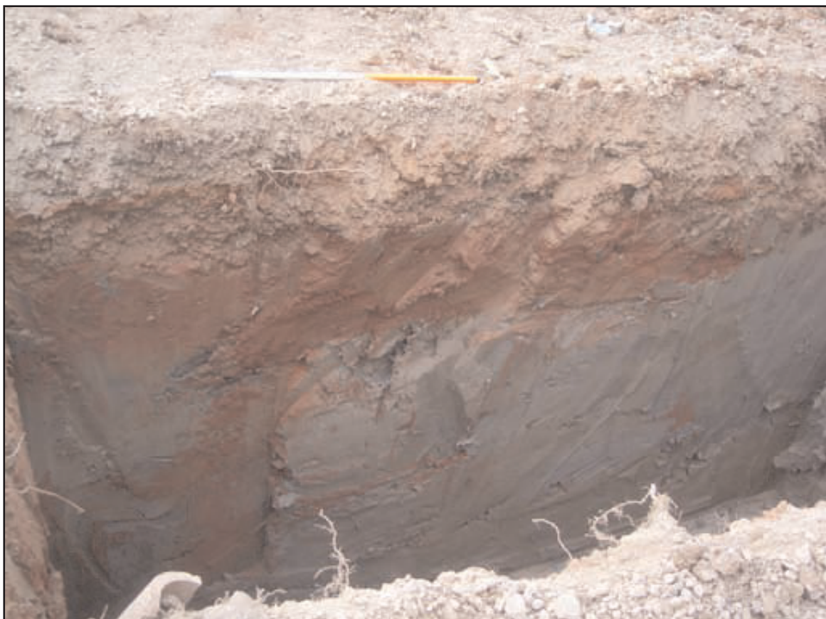
Plate 2 View of the southern section of the trench for the water tank, looking south
