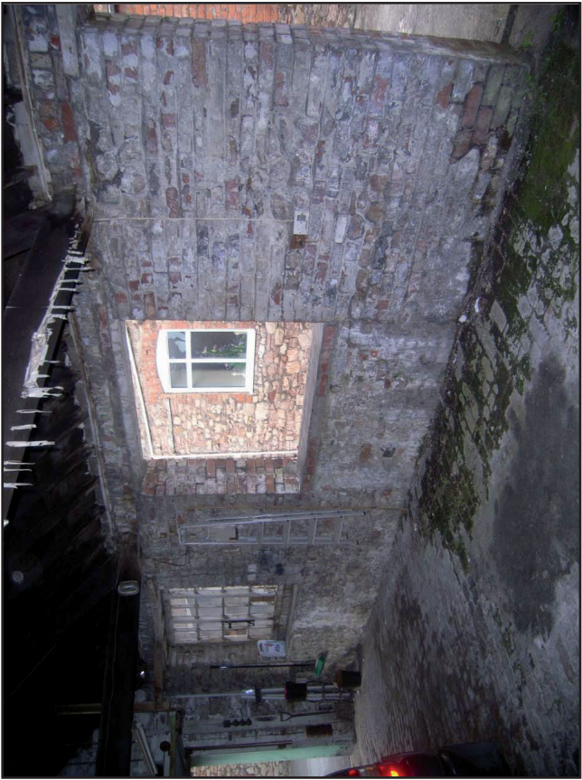
Plate 9 Interior of west wall, from north-east: note straight joint and area of brick walling
