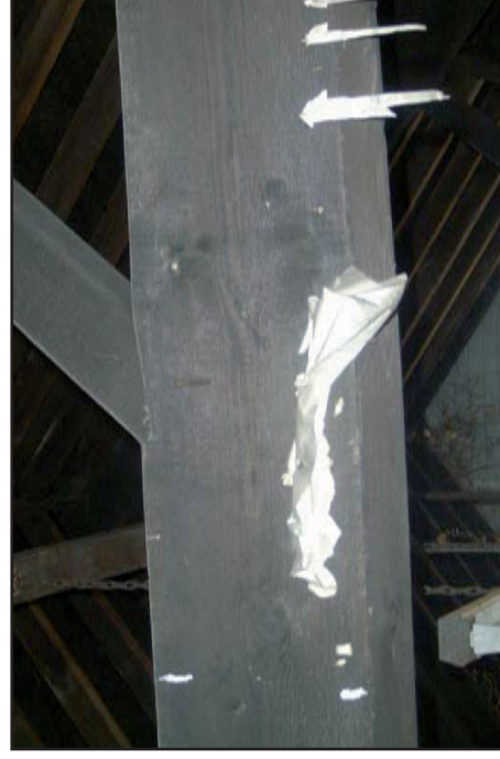
Plate 15 Northern roof truss: detail of carpenter's mark
