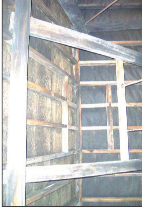
Plate 16 Underside of roof, showing site of possible former ventilator
