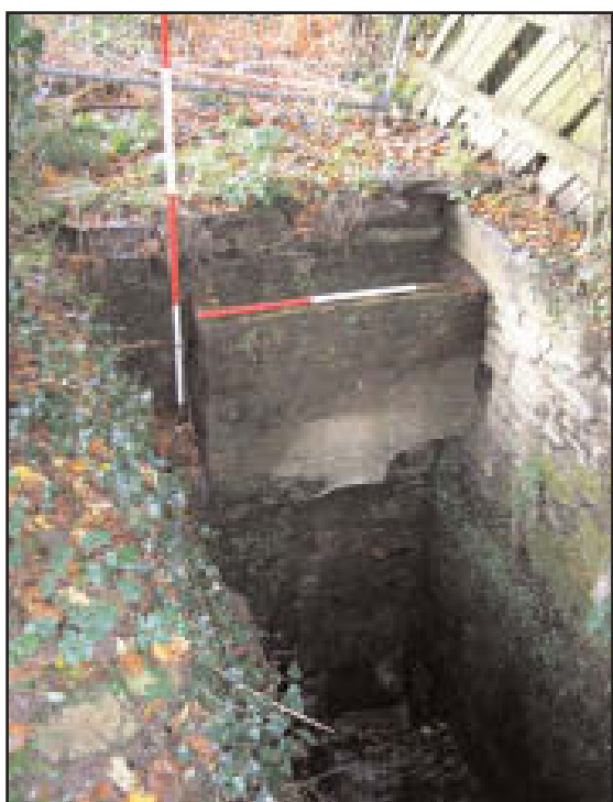
Plate 8 The brick and stone structure, looking south-west (scales 2m and 1m).
