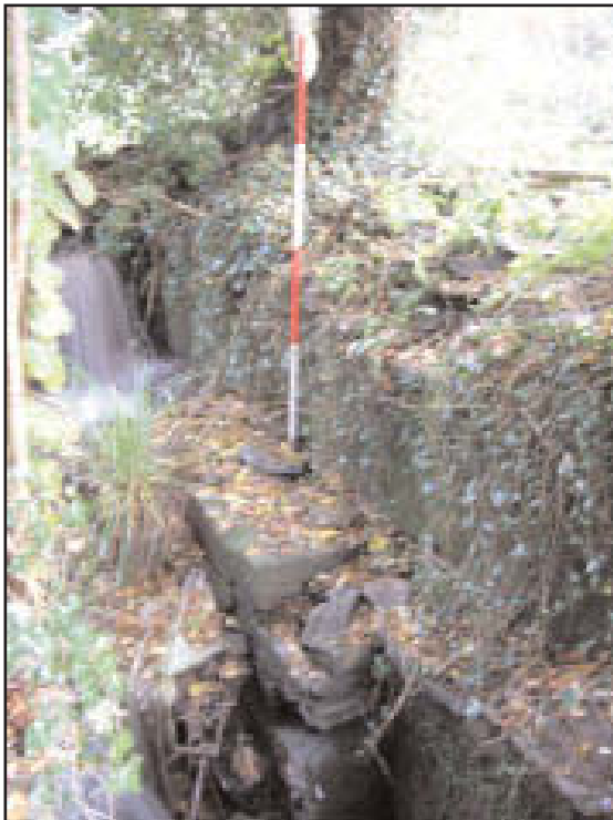
Plate 5 The east side of the waterwheel pit showing the east wall and offset, looking north-east (scale 2m)
