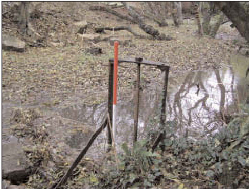
Plate 10 The sluice gate on the west end of the millpond, looking north-east (scale 1m)
