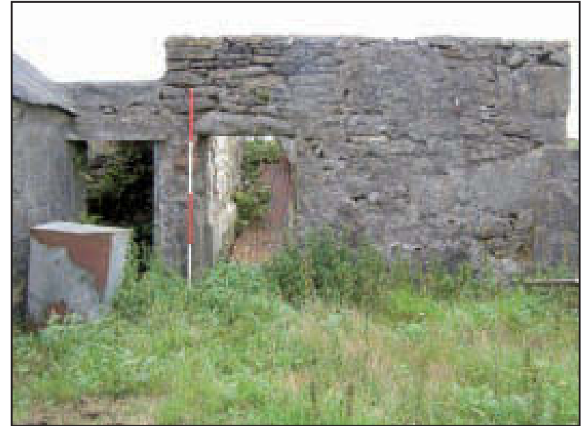
Plate 31 Building F: west elevation, looking east (scale: 2m)
