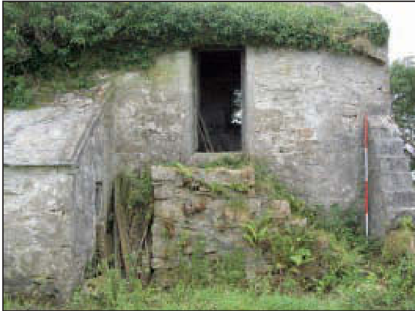
Plate 13 Building B: north elevation showing external stone staircase, first floor doorway and buttress on north-west corner, looking south (scale: 2m)
