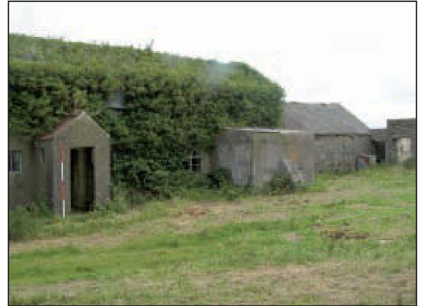
Plate 19 Building D: south elevation, looking north-east (scale: 2m)
