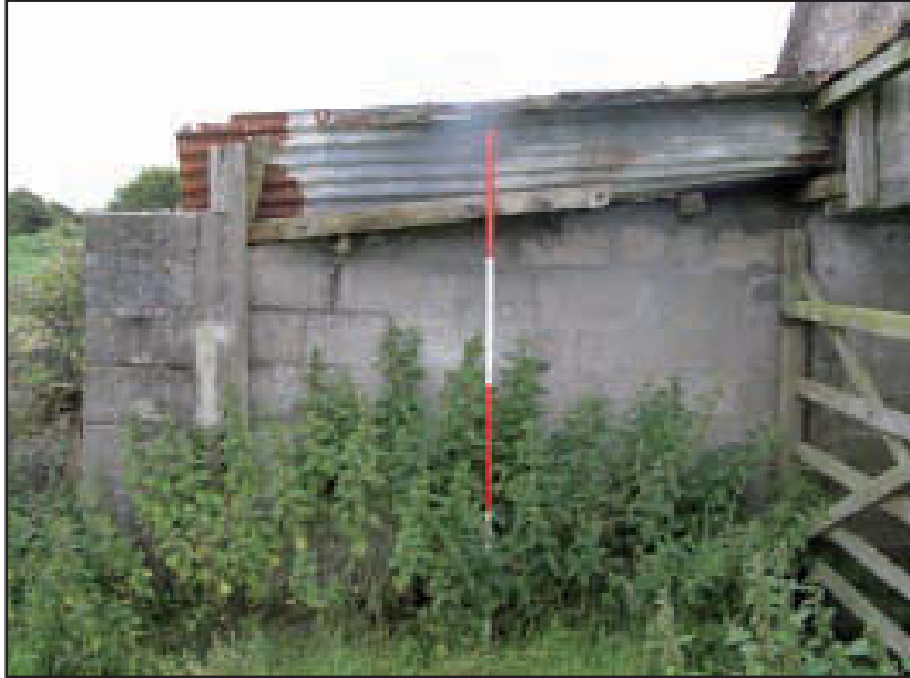
Plate 33 Building F: north elevation, showing concrete blocking, looking south (scale: 2m)
