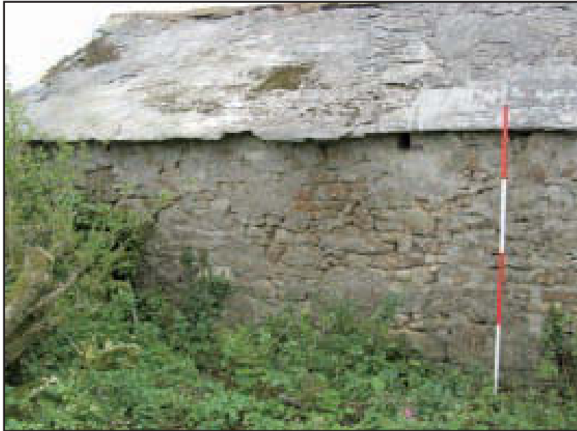
Plate 25 Building E: north elevation, looking south-east (scale: 2m)
