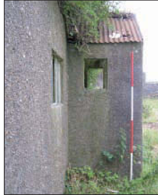
Plate 3 Building A: the porch, looking east (scale: 2m)
