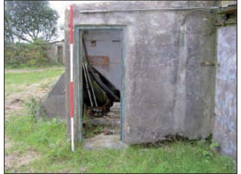
Plate 35 Building G: east elevation, looking west (scale: 2m)
