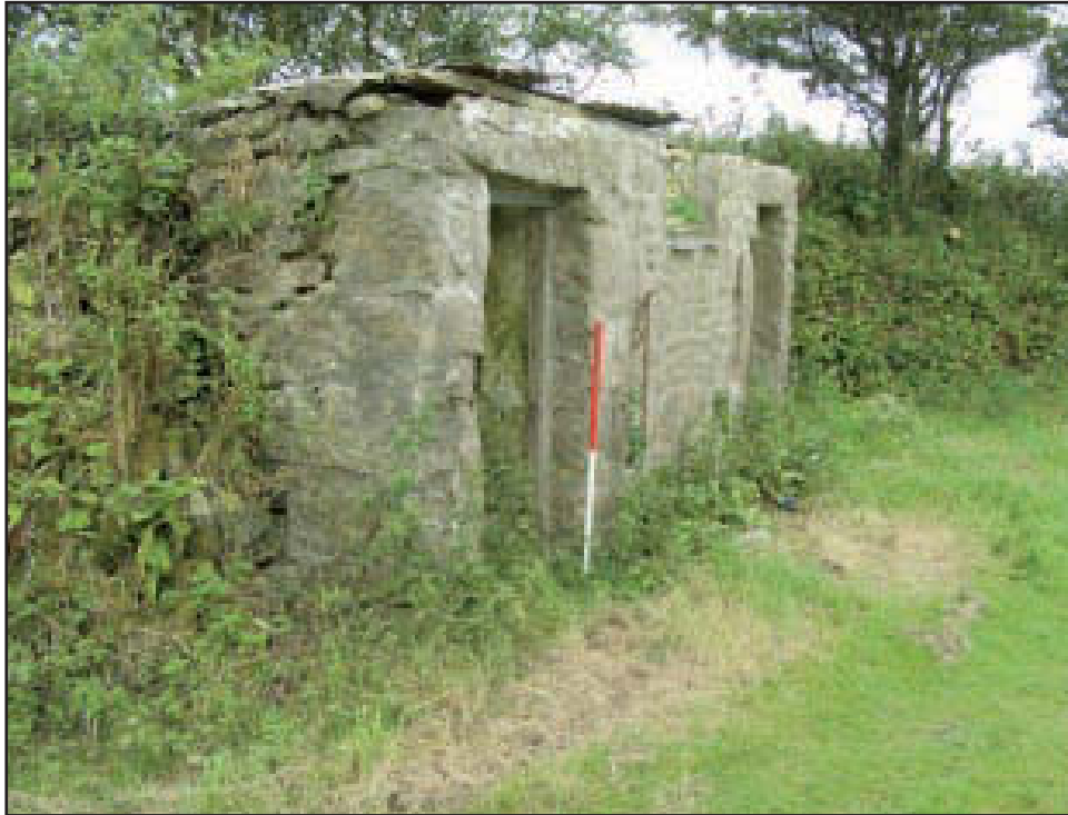
Plate 37 Building H: north-east elevation, looking west (scale: 1m)
