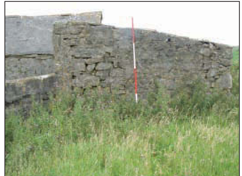
Plate 32 Building F: south elevation, looking north (scale: 2m)
