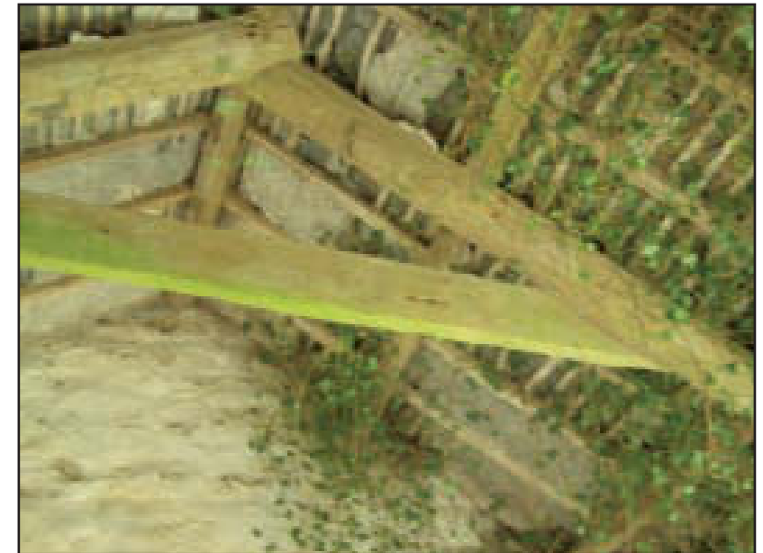
Plate 12 Building B: the roof showing A-frame and purlins (no scale)
