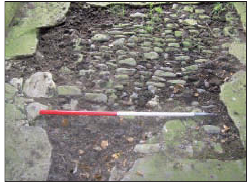
Plate 28 Building E: patch of cobbled floor showing through later concrete screed, looking east (scale: 1m)
