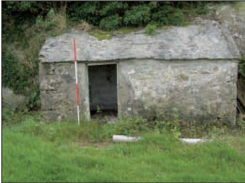
Plate 17 Building C: north elevation, looking south (scale: 2m)
