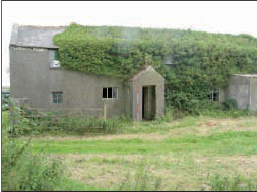
Plate 1 Building A: the south elevation, looking north (scale: 2m)
