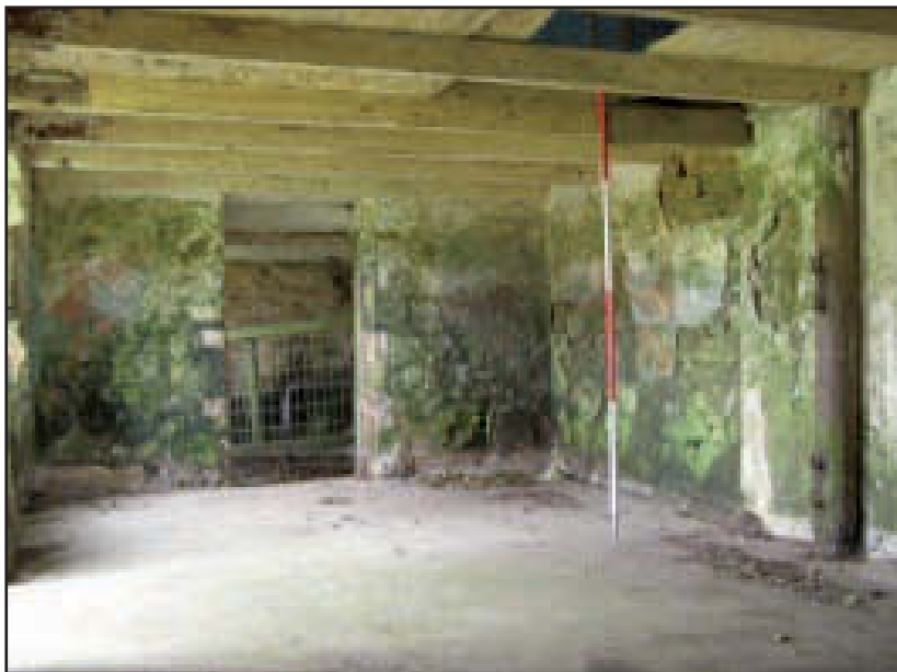
Plate 6 Building A: the ground floor showing the entrance to Building B; the ranging pole marks the position of the staircase, looking north-west (scale: 2m)
