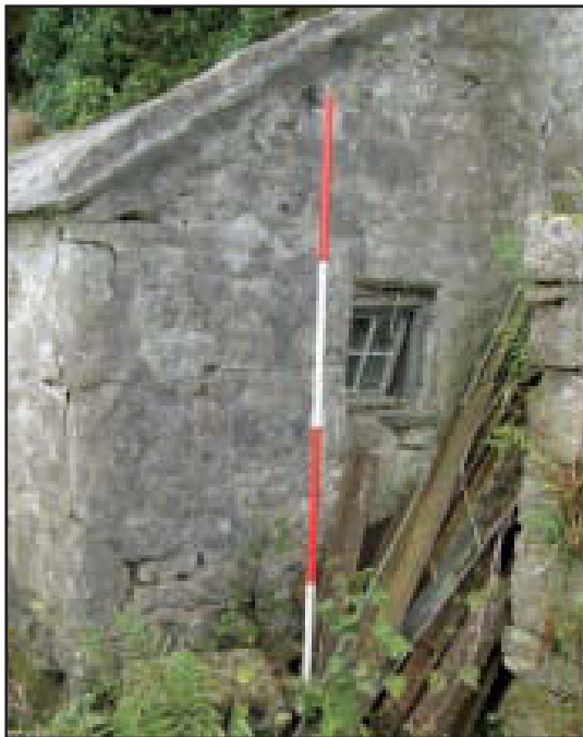
Plate 18 Building C: west elevation, looking south-east (scale: 2m)
