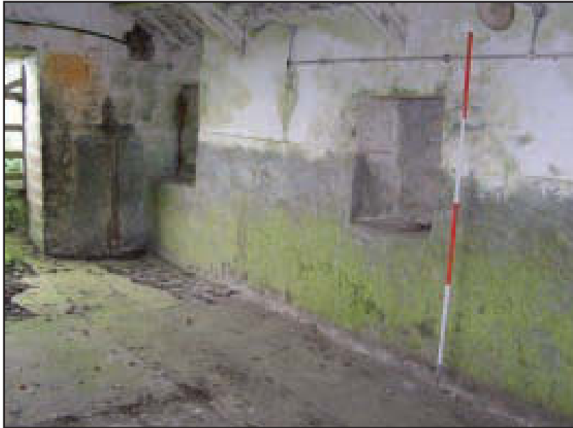
Plate 29 Building E: south wall showing blocked windows, looking south-east (scale: 2m)
