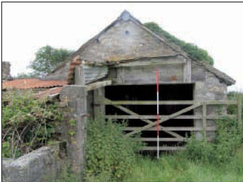
Plate 26 Building E: east elevation, looking west (scale: 2m)
