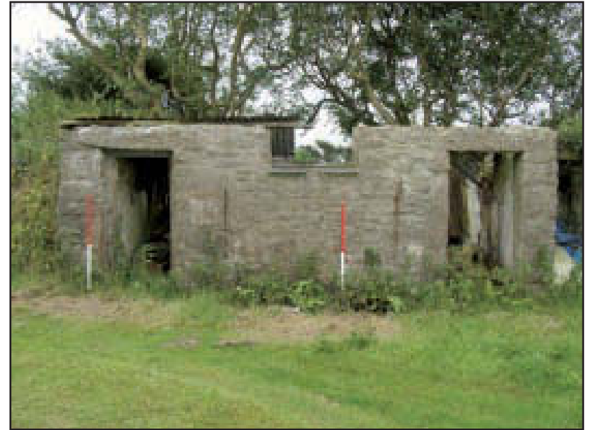
Plate 36 Building H: north-east elevation, looking south-west (scales: 1m)
