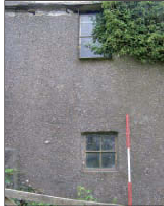
Plate 15 Building B: windows in south elevation, looking north (scale: 2m)
