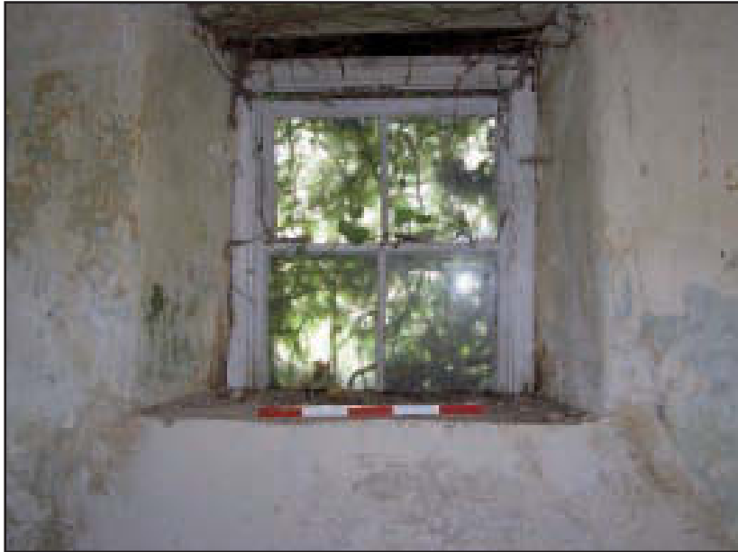
Plate 5 Building A: first floor sash window, looking south (scale: 0.5m)
