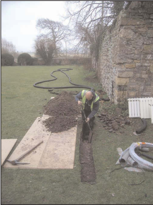
Plate 6 Manual excavation of cable/pipe trench in progress across the lawn of the outer court (looking south)
