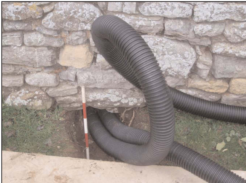
Plate 5 East-side of garden wall, showing hole made for plastic pipe to/from heat pumps (looking west)
