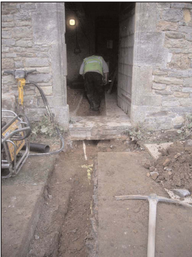
Plate 8 Doorway into store room at west-end of farmhouse. Note existing electric cable (within white plastic sleeve) passing under door sill
