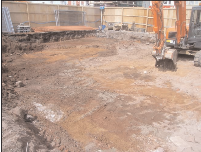
Plate 4 Reduced level excavation of the western side of site, prior to foundation excavation, looking west
