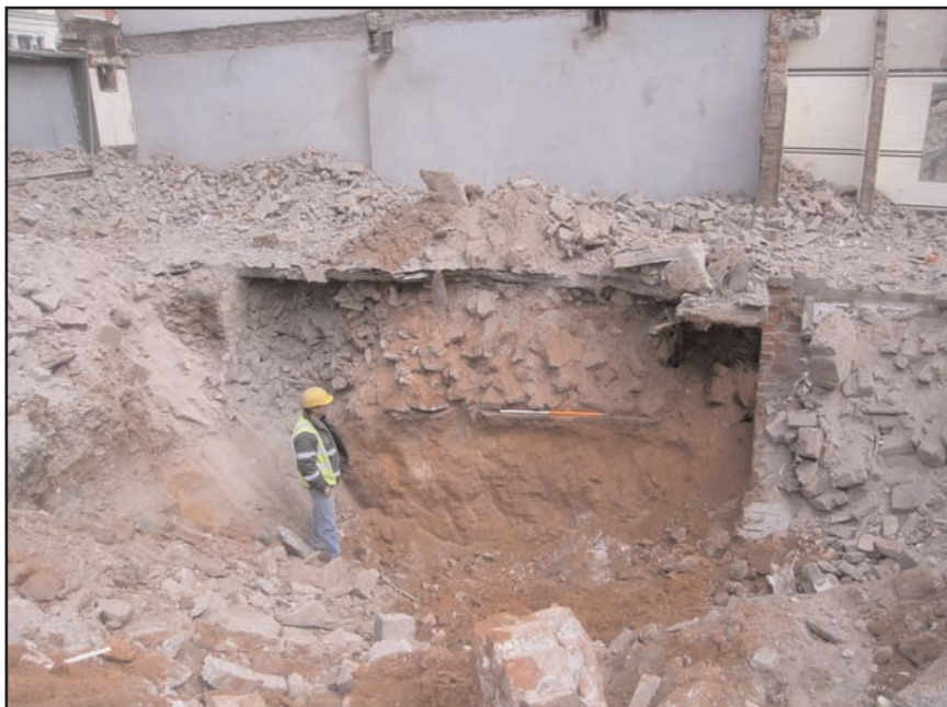
Plate 2 Detail of the main cellar during demolition, also shows the original floor level outside the cellar area and the cellar back- wall continuing to the north-east, 1m scale
