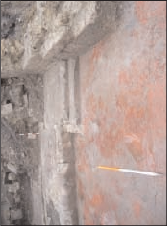
Plate 5 Looking north, at pair of stone steps (112) within the western domestic wing
