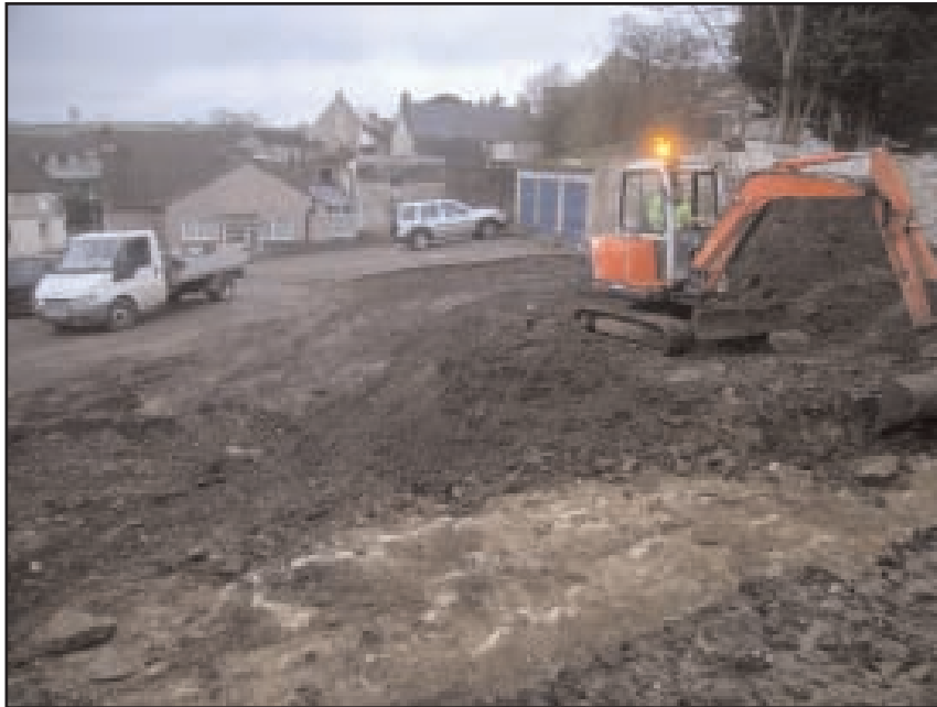
Plate 3 The natural lias bedrock being exposed during ground reduction work – looking south
