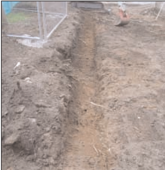
Plate 5 General view of foundation trench excavation for the extension, looking west
