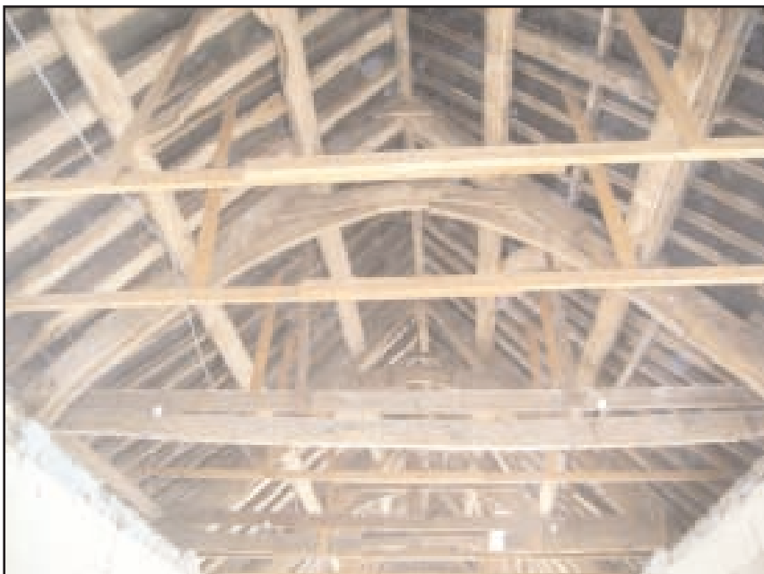
Plate 12 The timber frame supporting the roof of Room G1, looking east
