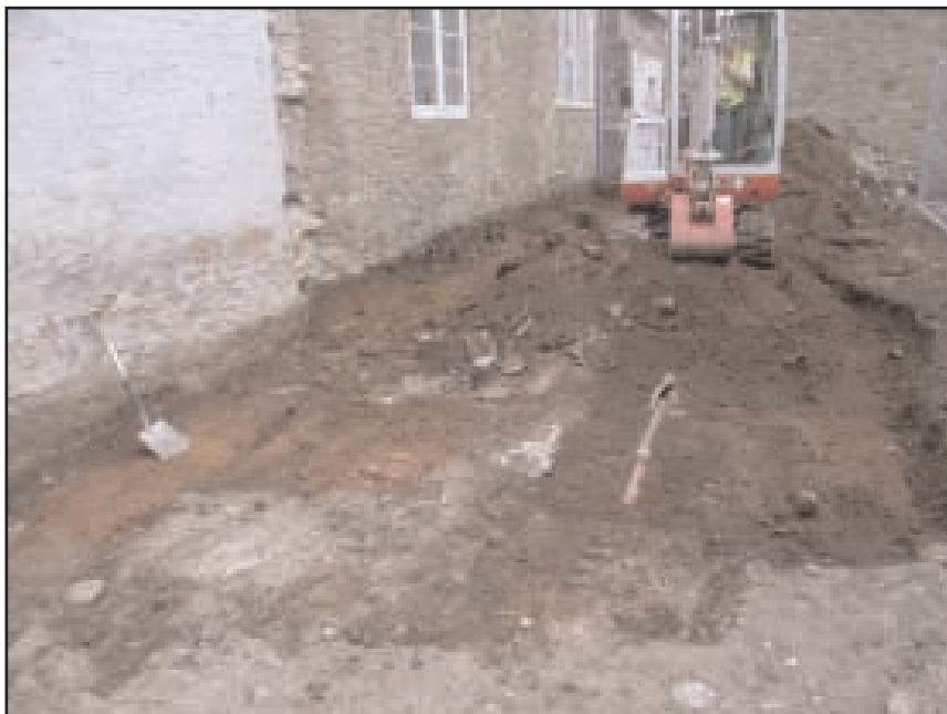
Plate 2 General view of the reduced level excavation with the footings of the demolished outbuilding and a modern ceramic service pipe in fore- ground, looking ENE
