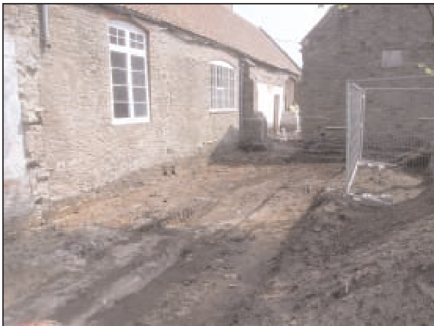
Plate 3 General view of the reduced level excavation, looking ENE
