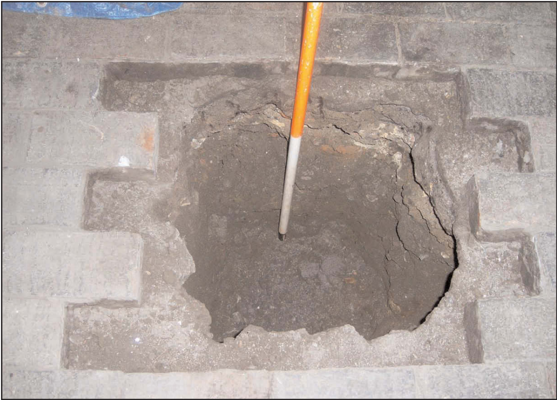
Plate 1 Test pit during excavation, looking west
