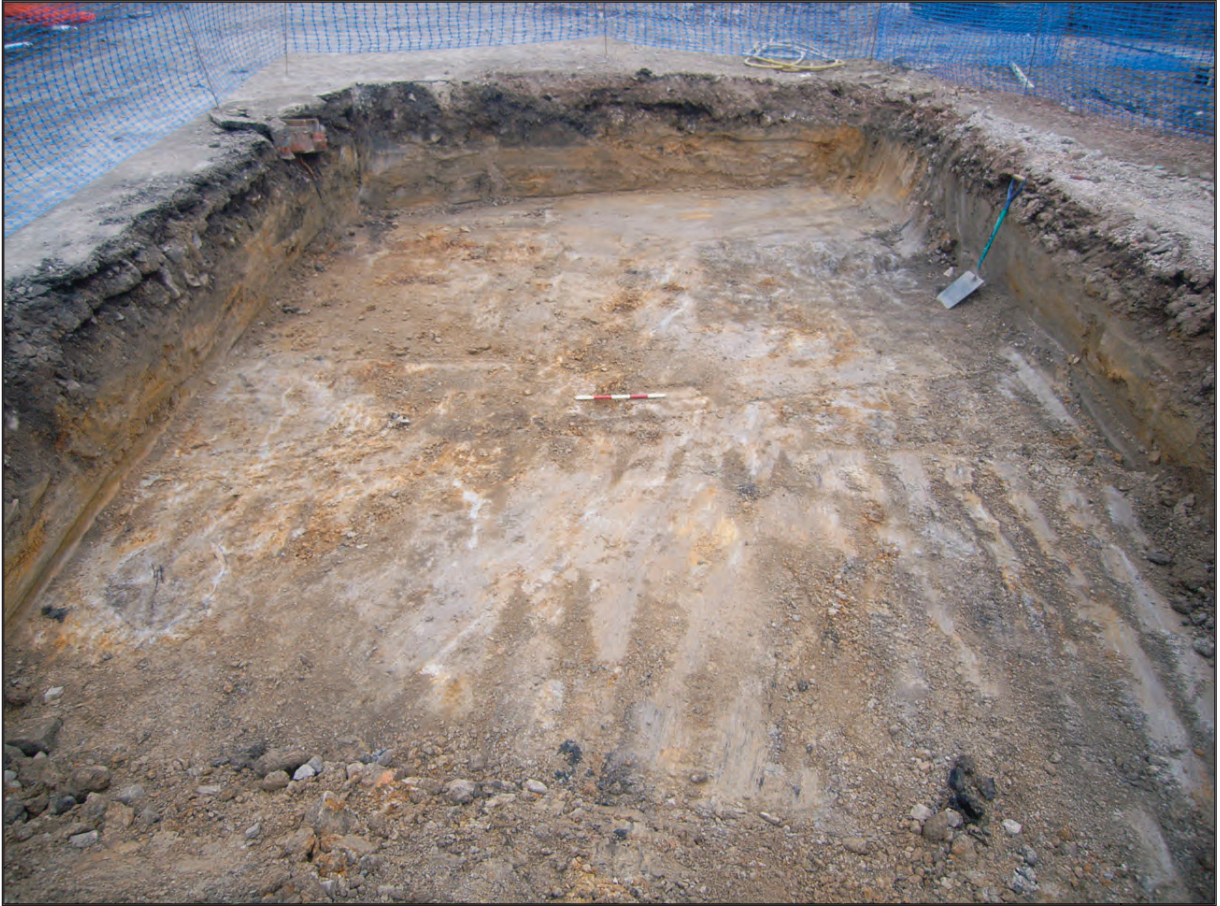
Plate 3 Attenuation tank area, excavated down to natural yellow clay, looking south-east
