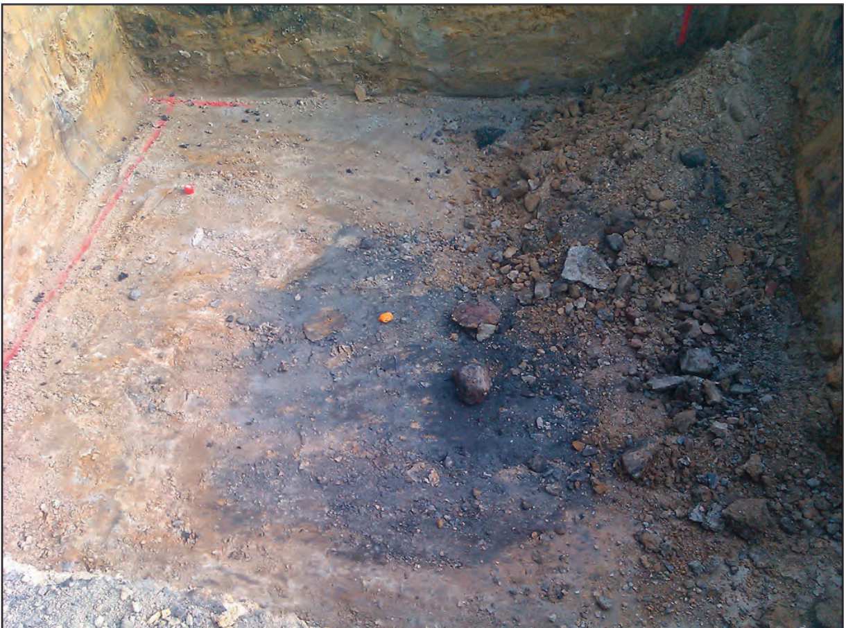
Plate 4 Top of the coal shaft before consolidation, looking north
