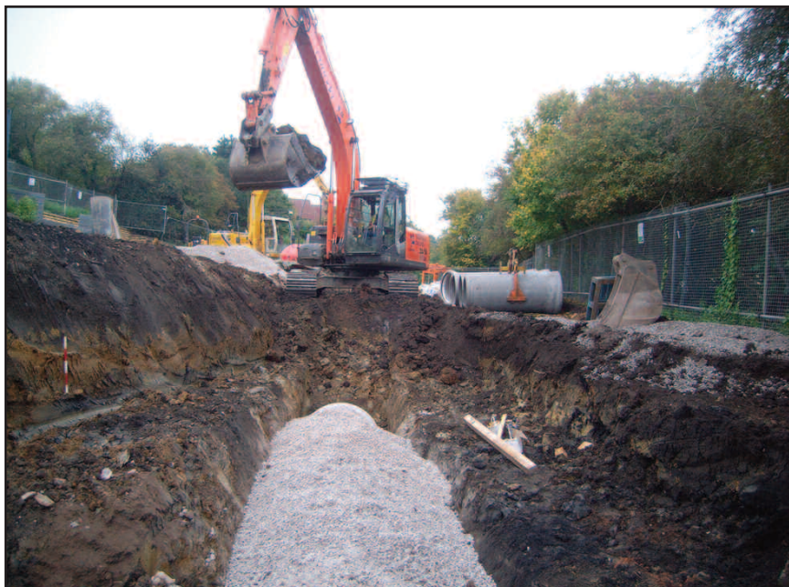
Plate 9 Digging the 'attenuation tunnel', viewed from the west
