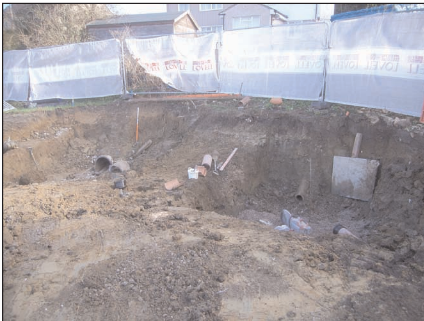
Plate 2 Excavation to connect new drainage pipe with existing services and install manhole access chambers, looking north- north-east, scale 1m
