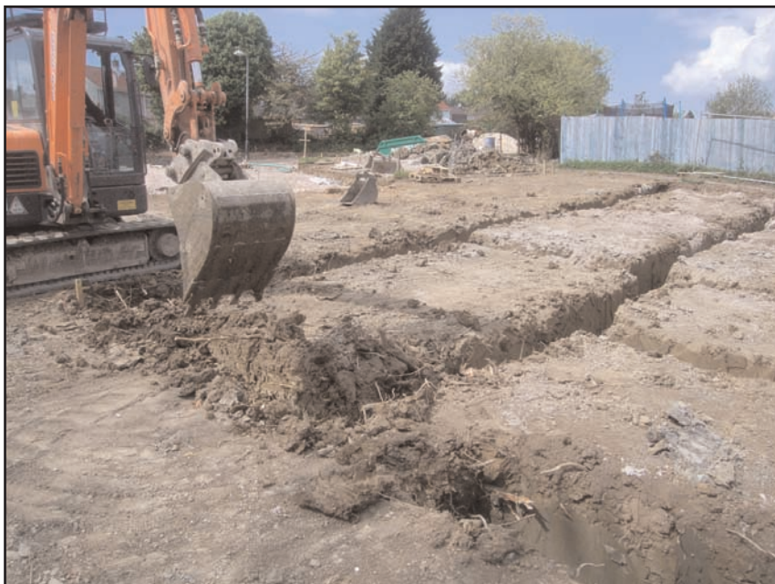
Plate 6 General view of the excavation of footings for Plot C, looking north, 1m scale
