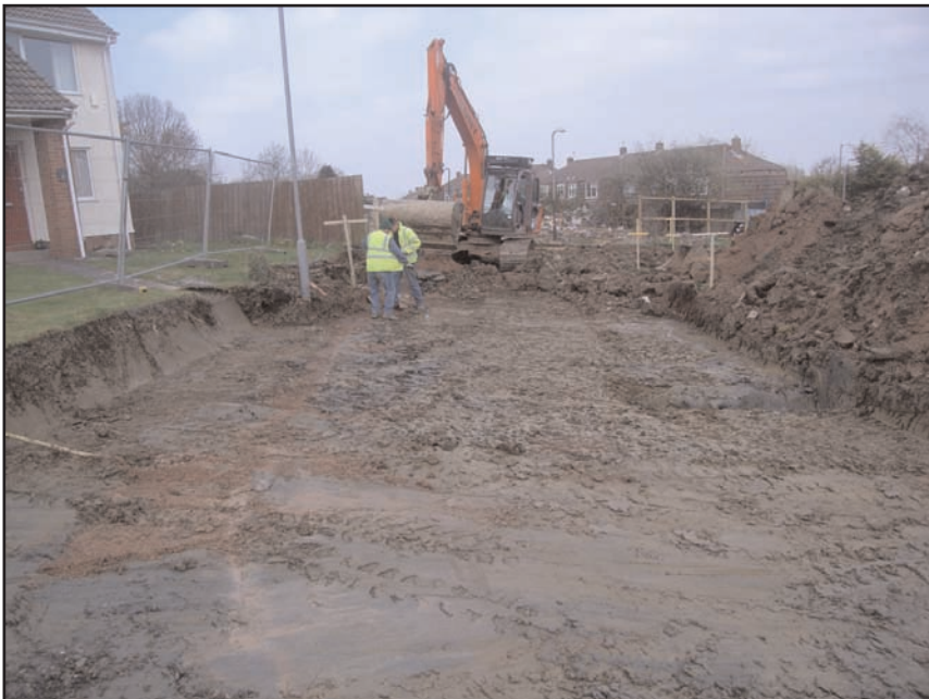
Plate 2 General view of the excavation of the site road, looking north-east
