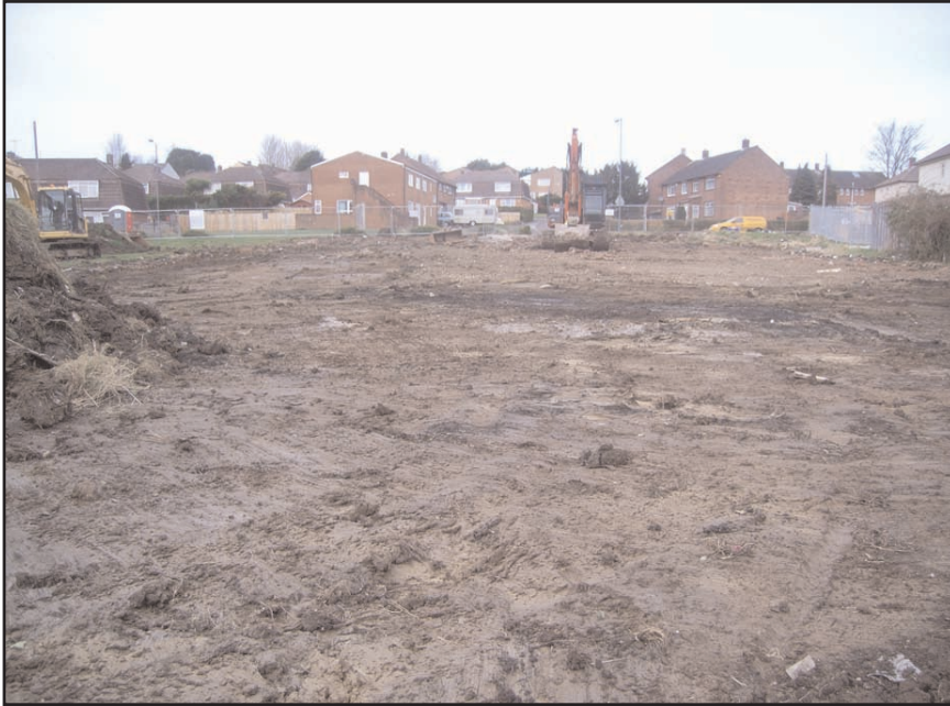
Plate 1 General view of the topsoil stripping, looking east
