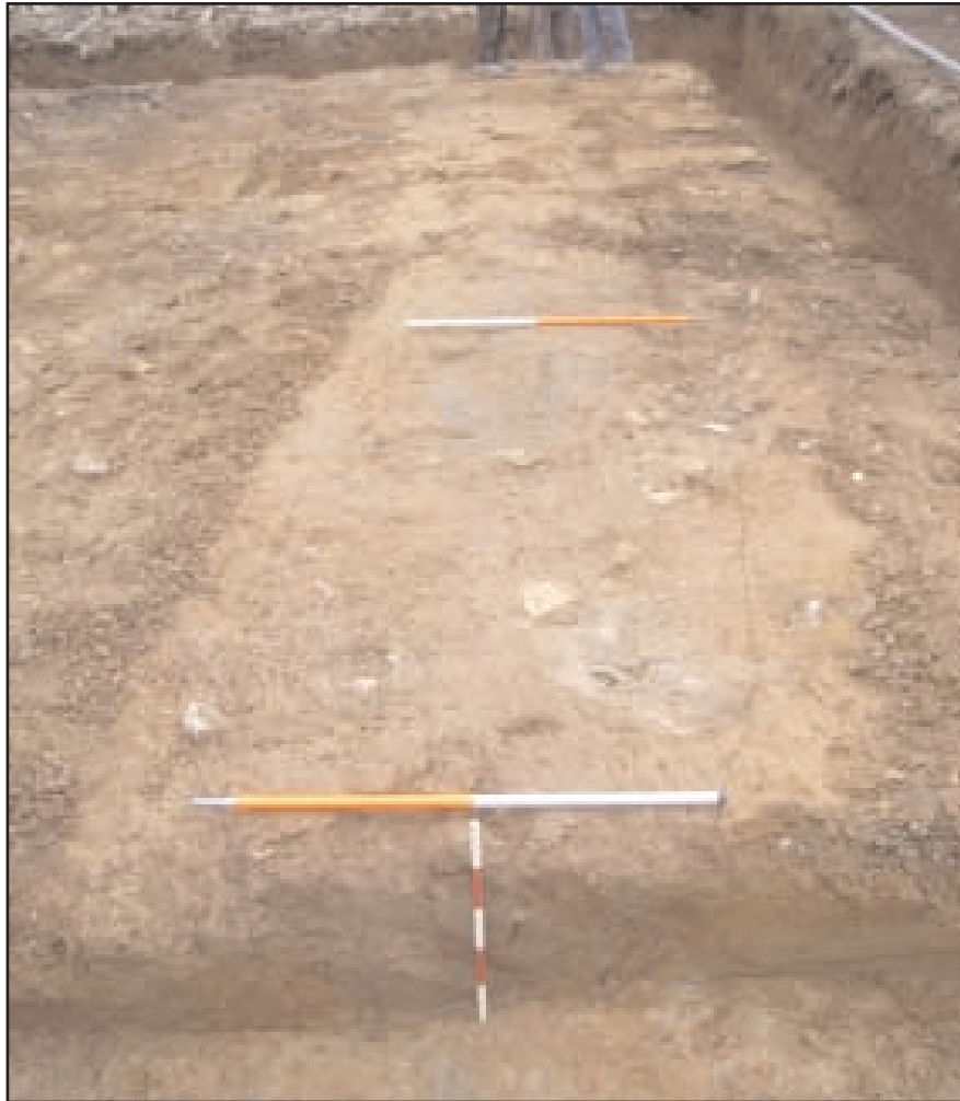
Plate 3 Foundation trench excavated through cut [105] and fill (106) looking east, scales 1m & 0.5m in foreground
