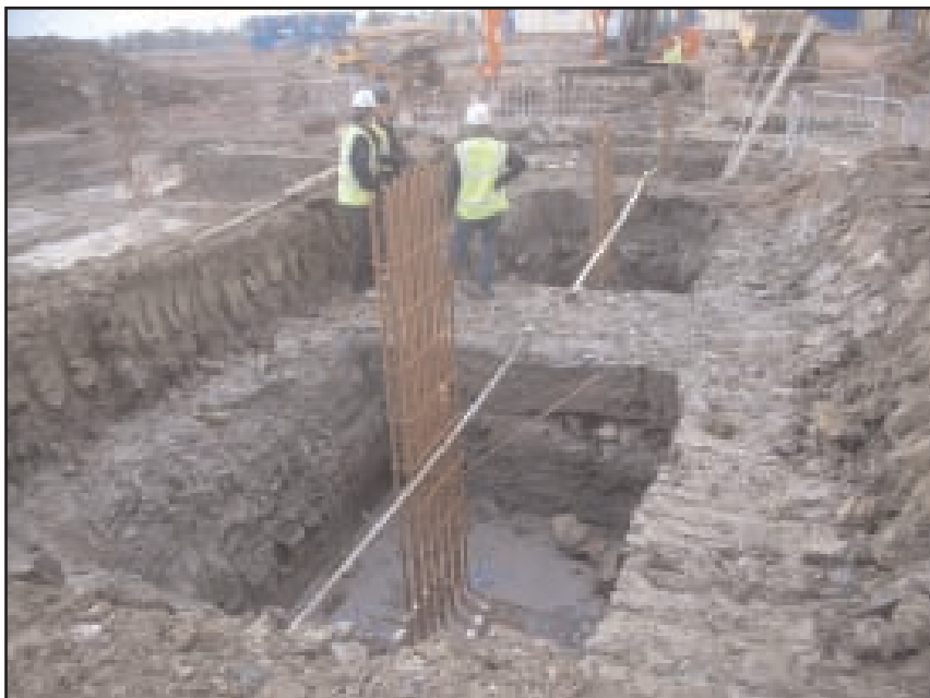
Plate 6 Foundation excavation for the new hospital building after initial reduced level excavation, looking east
