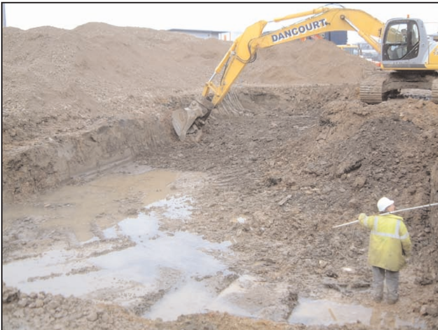
Plate 8 Excavation of pit for attenuation tank, looking north & north-west
