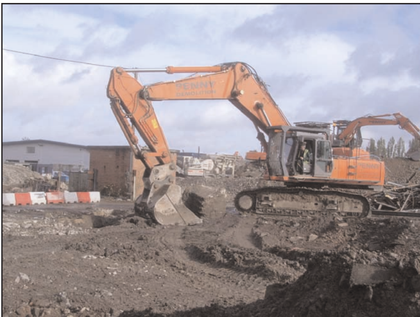
Plate 3 Excavation of concrete pier bases belonging to former Countrywide Farmers depot
