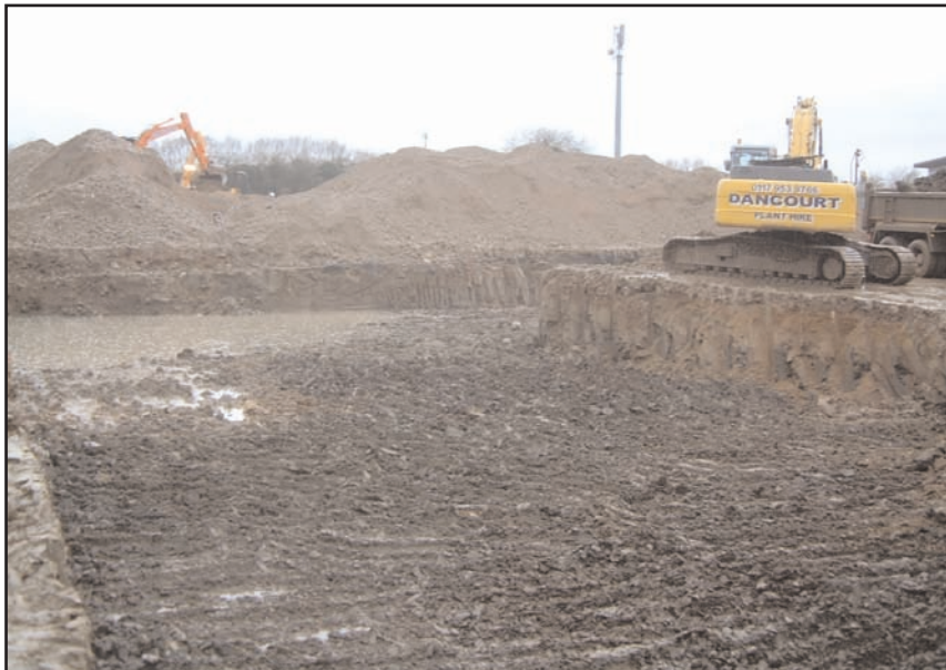
Plate 9 Excavation of pit for attenuation tank, looking north & north-west
