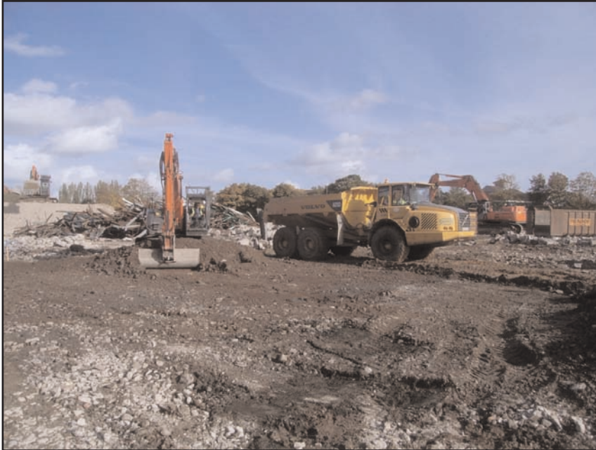
Plate 1 Ground reduction (‘proofing’) in progress – looking north-east across site
