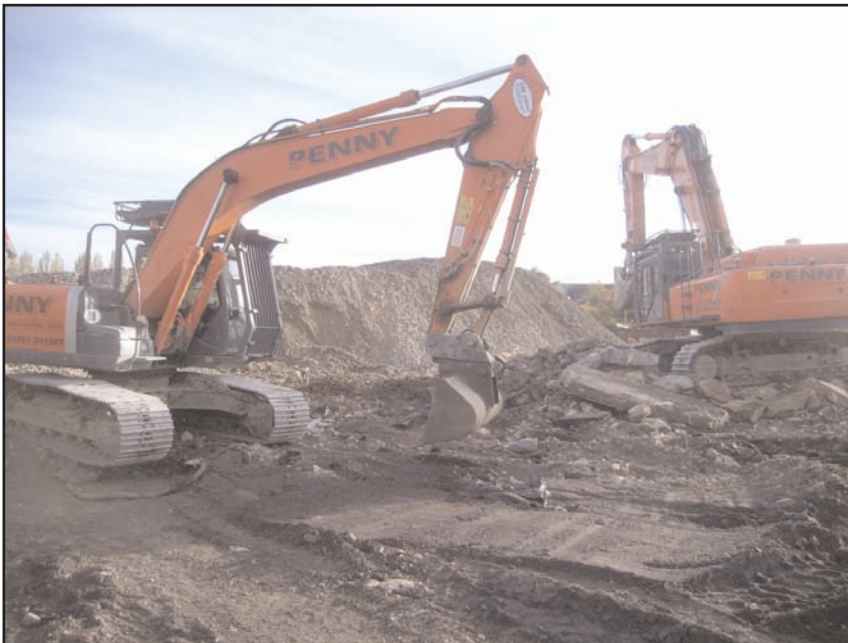
Plate 2 Ground reduction (‘proofing’) in progress – looking north-east across site
