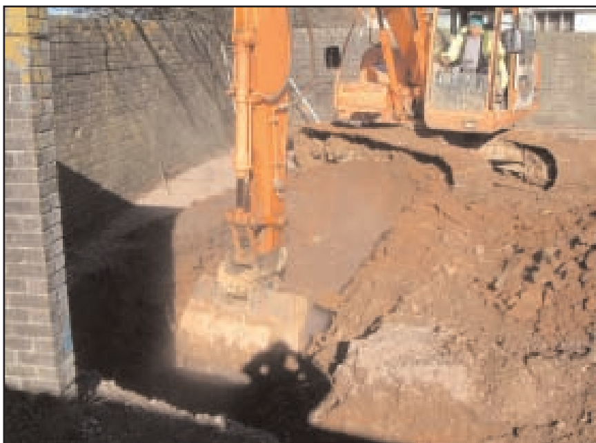
Plate 3 Excavation of 2.5m deep trench for diverted mains sewer
