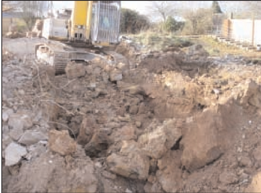
Plate 1 Mechanical removal of foundations belonging to the former care home
