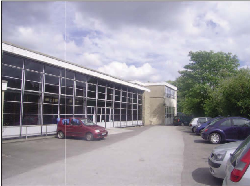
Plate 4 Extension to Hayesfield Lower School, built in 1960, with later additions in the background, viewed from the south- west
