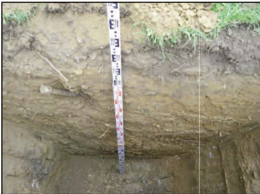
Plate 8 Geotechnical trial pit 5
