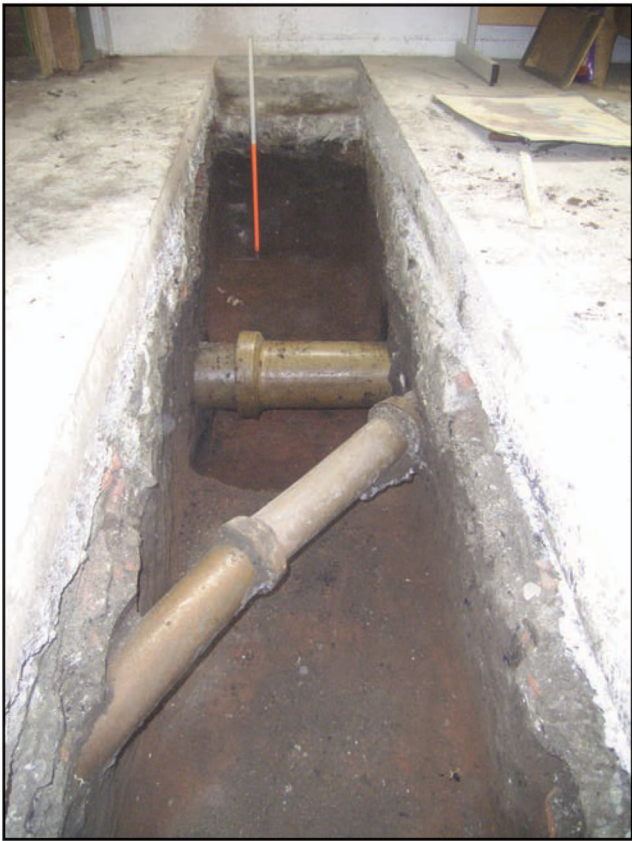
Plate 1 Test Pit 3 as excavated, exposing brick floor below concrete, looking north-west, Scale 0.5m
