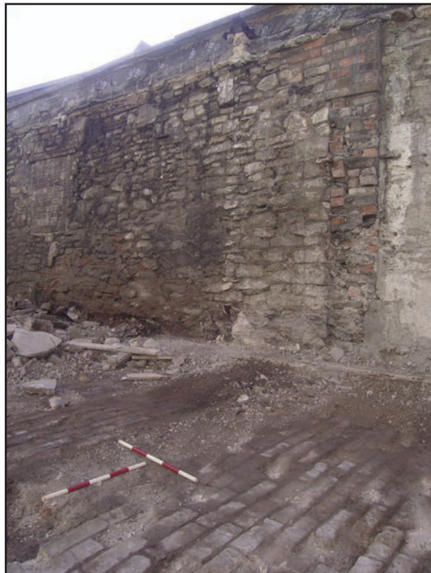
Plate 3 Detail of former wall cutting the brick surface and the scar of where it butted the property boundary, looking south-west, 2 x 0.5m scales
