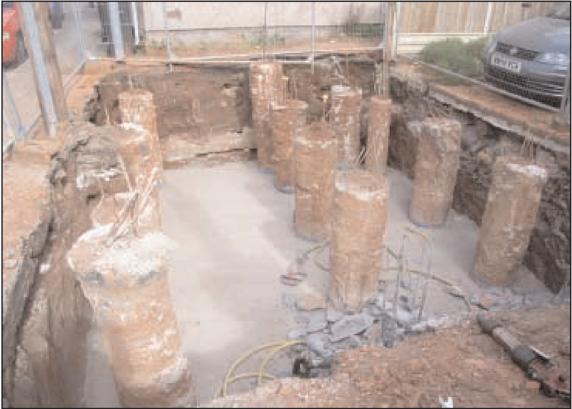
Plate 1 Northern half of site after ground reduction, looking north
