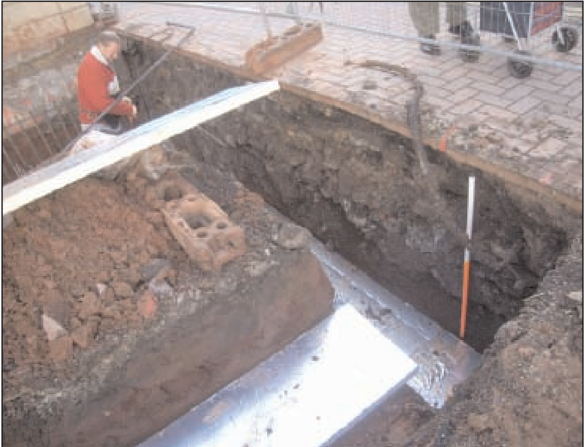
Plate 2 Southern edge of site showing remains of terraced housing footings, looking south-east towards North Street
