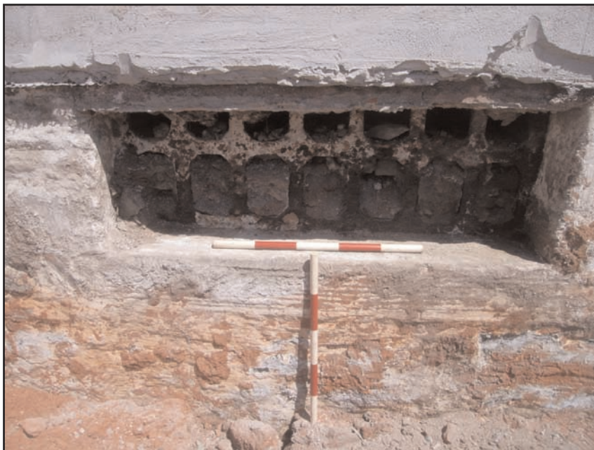
Plate 8 Detail of opening 116 as exposed, looking north- east, 0.5m scales
