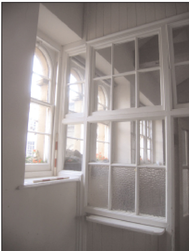
Plate 3 Detail of the north-west end of the partition built into a window bay (Classroom 1) looking east, 2 x 0.5m scales
