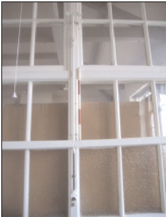
Plate 6 Detail of device for opening upper window panes (Classroom 1) looking east-north-east, 0.5m scale
