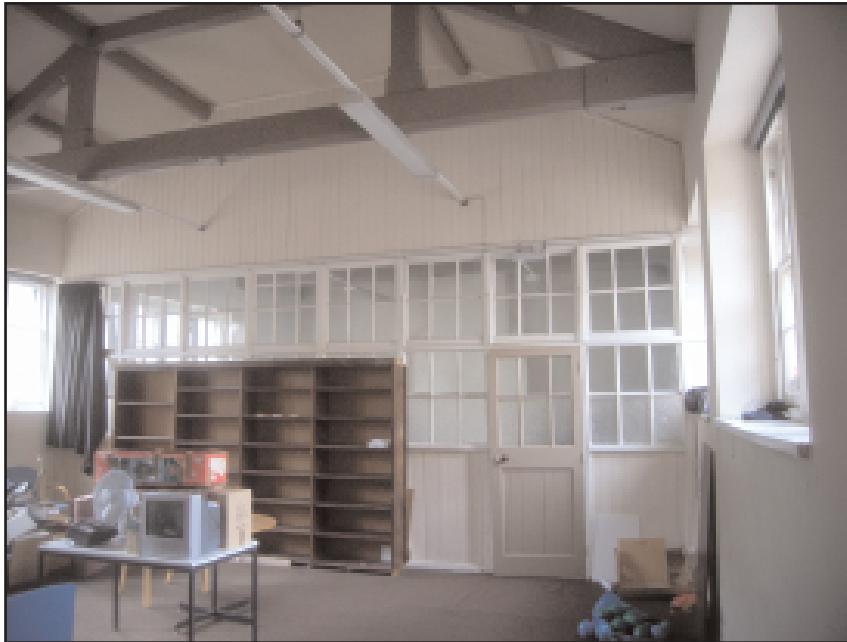
Plate 5 Overall view of partition in Classroom 2, looking south-south-west, 0.5m scale
