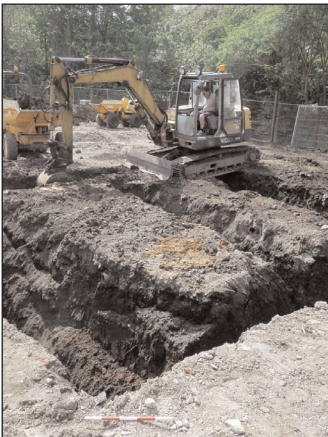
Plate 3 Excavation of Trench 5 in progress, looking SW, scale 0.5m
