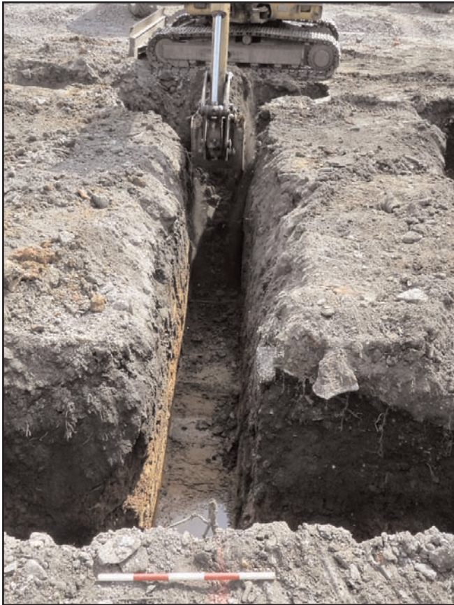
Plate 1 Completion of Trench 3, looking south, scale 0.5m
