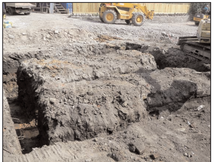
Plate 4 General view across the footings as excavated, looking south-east
