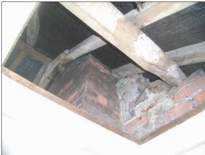
Plate 53 View through loft hatch on first floor (original Masons Arms)
