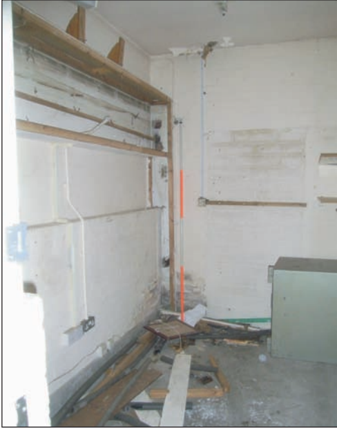
Plate 37 General view across Office on ground floor (1950s), from the north-east
