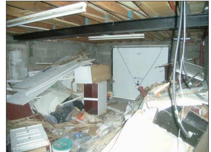
Plate 36 General view across Garage on ground floor (1979/80), from the south-east
