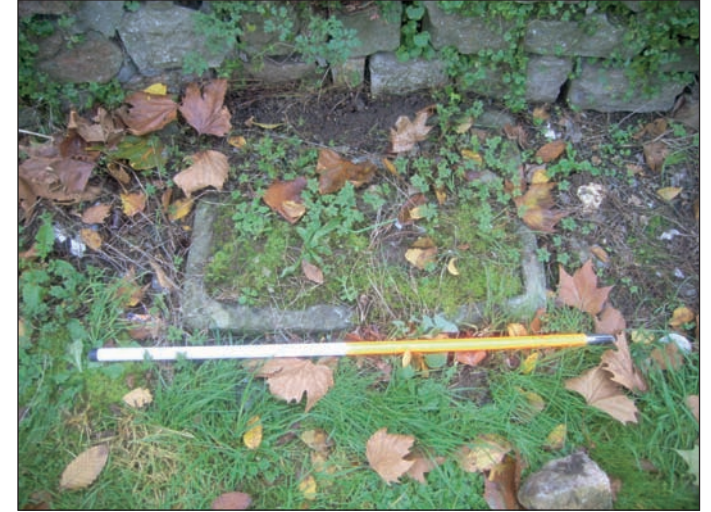
Plate 15 Detailed view of buried stone-trough immediately outside north flank of study area, from the north
