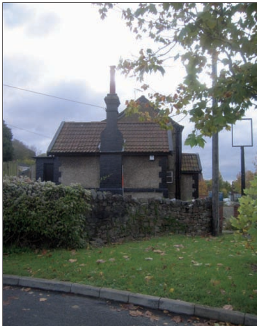
Plate 4 General view of part north-east elevation (the original Masons Arms), from the north-east
