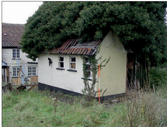
Plate 11 General view of external WC block (20th century), from the south
