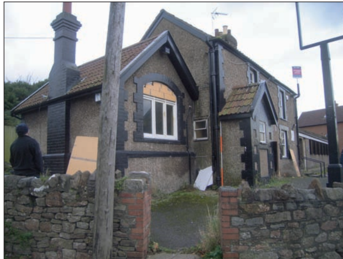
Plate 2 General view of part north-west and north-east elevations (the original Masons Arms), from the north
