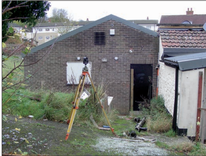
Plate 8 General view of part north-east elevation (1950s), from the north-east
