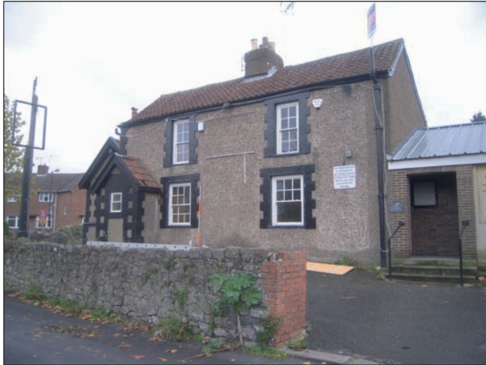
Plate 1 General view of part north-west elevation (the original Masons Arms), from the west
