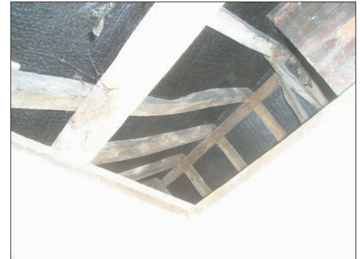
Plate 54 View through loft hatch on first floor (original Masons Arms)
