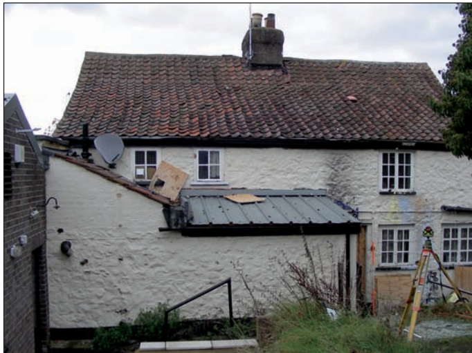
Plate 10 General view of part south-east elevation (original Masons Arms), from the south-east
