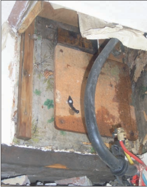
Plate 25 Detailed view of exposed wallpaper on south-west wall of Smoking Room on ground floor, from the north-east
