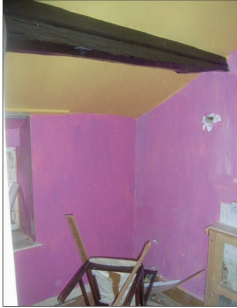
Plate 50 General view across Kitchen on first floor (original Masons Arms), from the north
