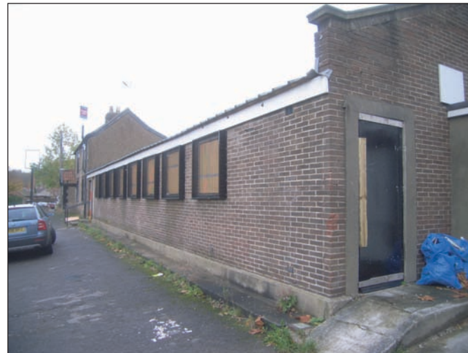
Plate 5 General view of part north-west elevation (1950s), from the south-west
