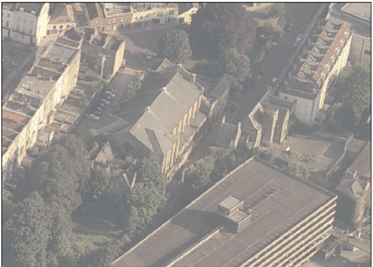
Plate 5 Aerial photo, looking north, taken prior to the demolition of the Presbytery and Saint Catherine's Convent (August 2005)
