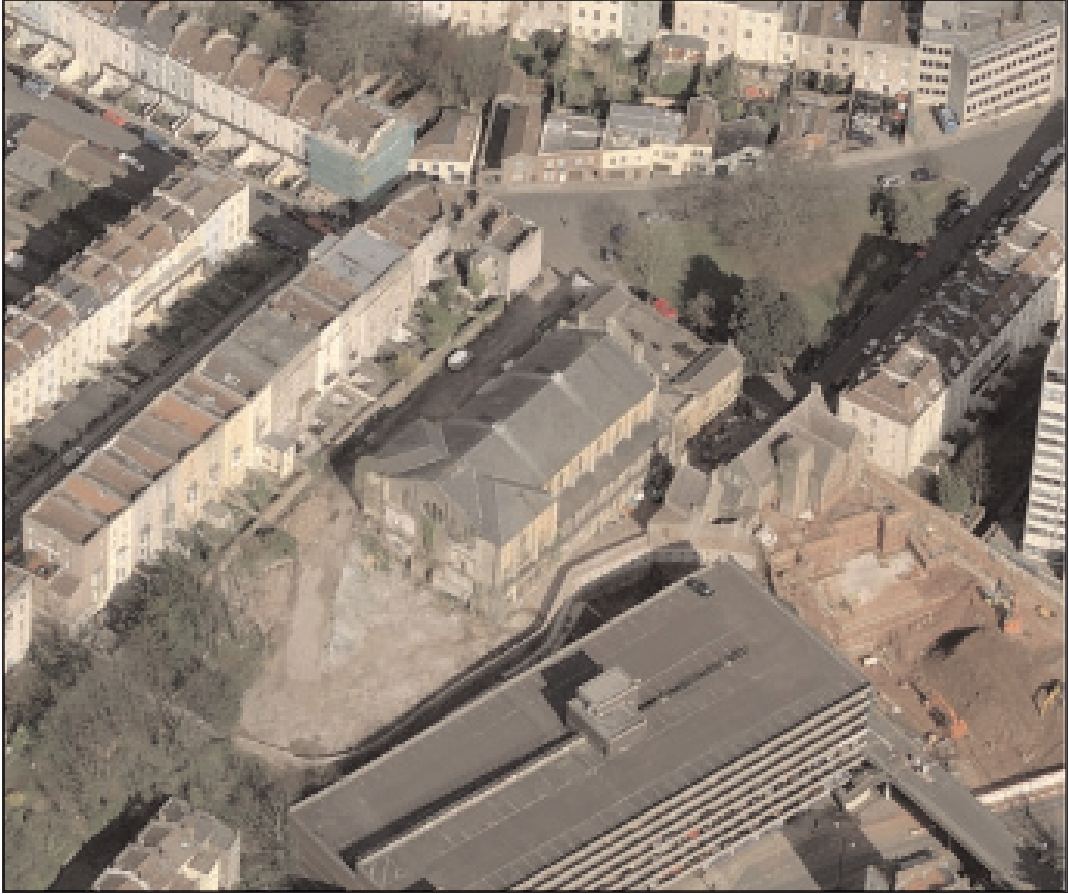
Plate 6 Aerial photo, looking north, taken after the demolition of the Presbytery and Saint Catherine's Convent (March 2008)
