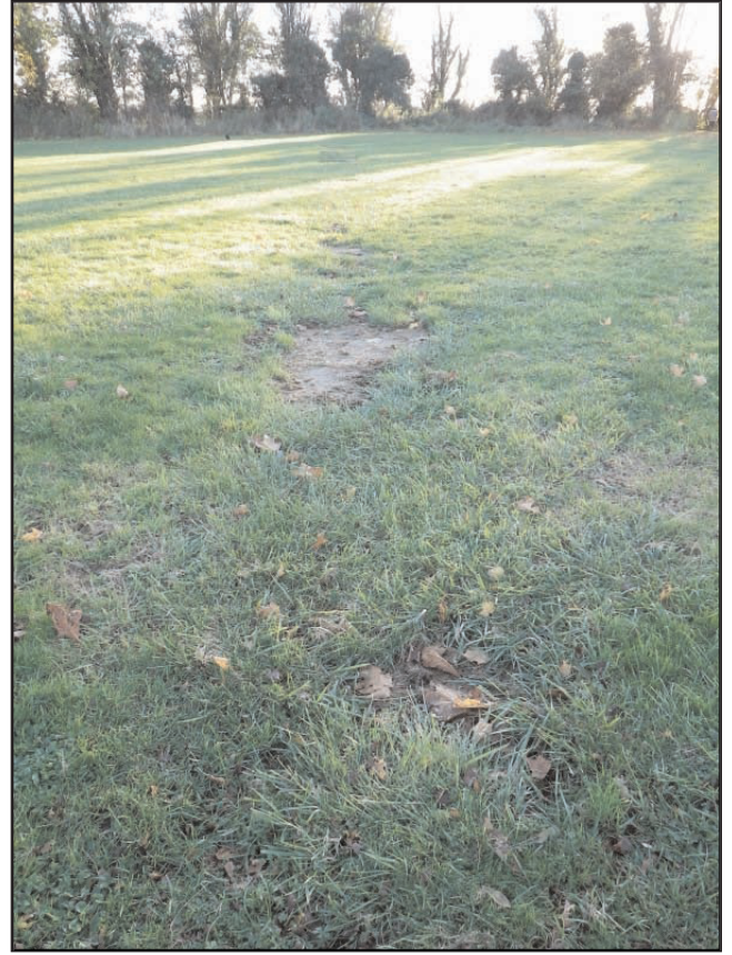
Plate 2 Concrete blocks running north-south on the west section of the site, looking south
