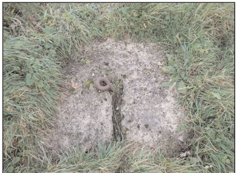
Plate 6 Central concrete balloon tethering block, looking east
