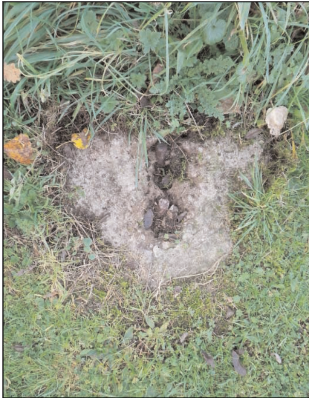
Plate 4 Concrete balloon tethering blocks, looking east
