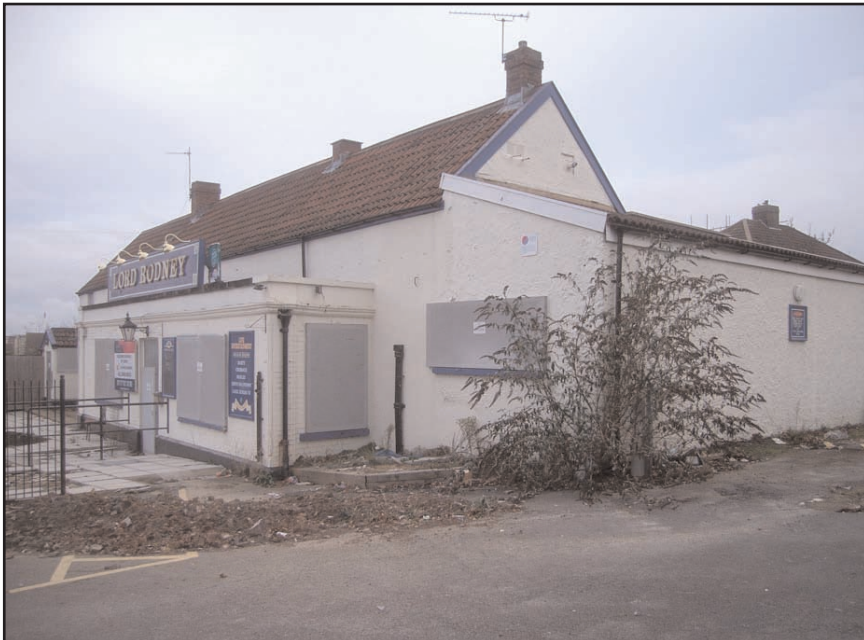
Plate 2 Southern frontage of Lord Rodney showing 1911 extension, looking north- east
