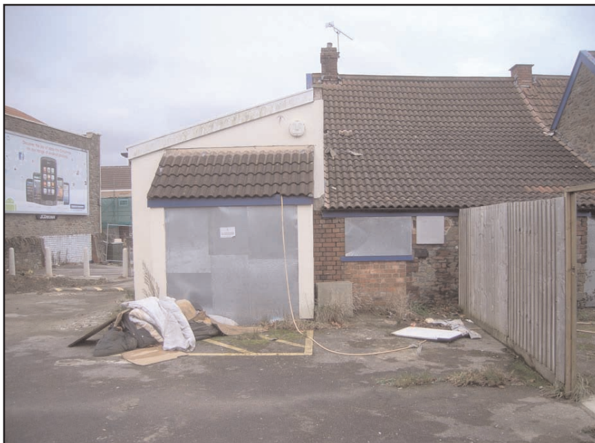
Plate 5 Looking south towards former stable block and former cart shed
