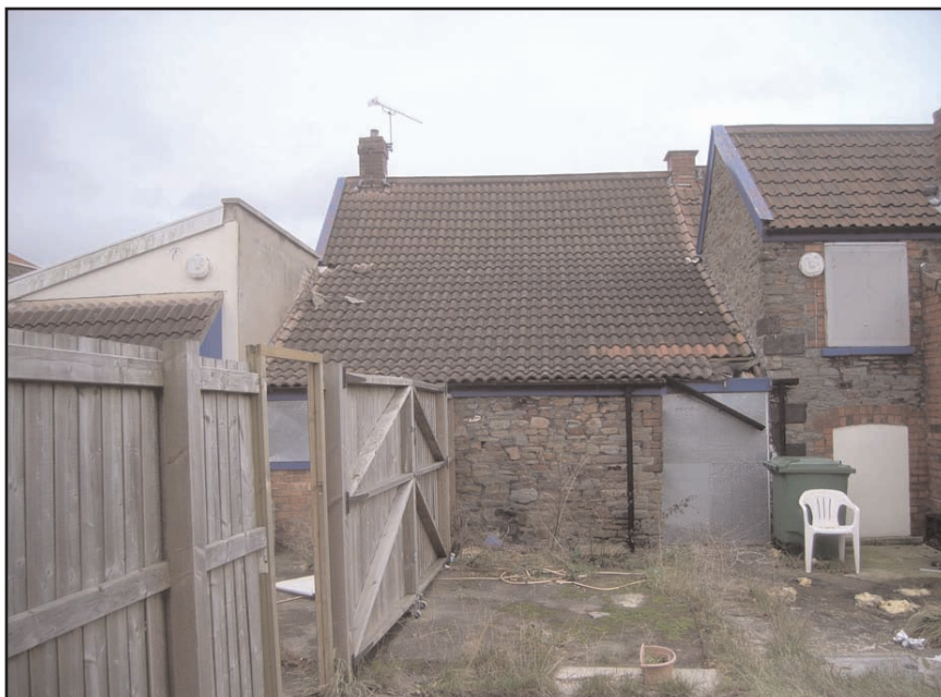
Plate 6 Looking south at former entrance to stable block
