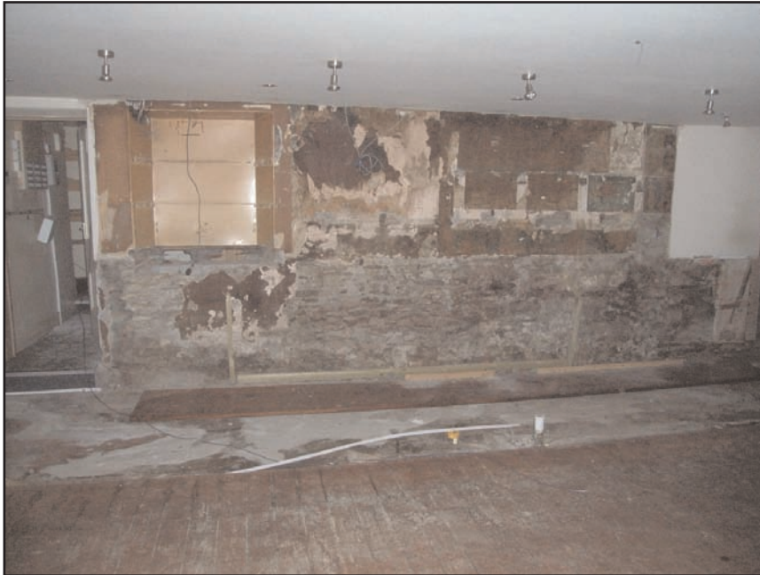
Plate 13 Southern face of central wall, showing blocked window, looking north
