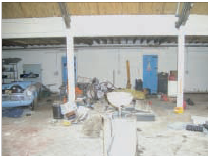
Plate 13 Internal space of the central block, Room 9, looking north
