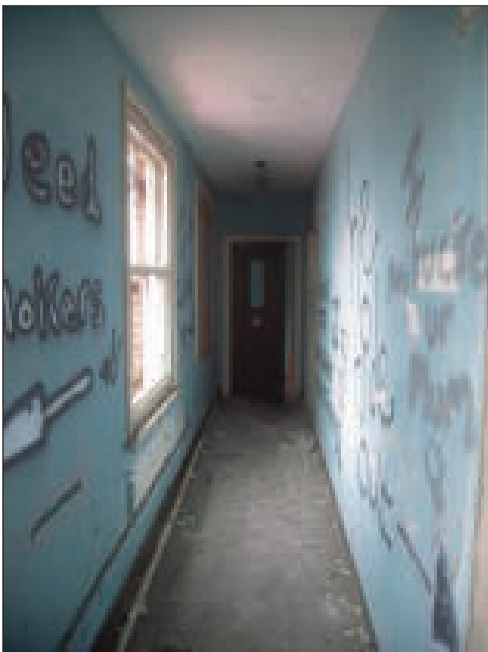
Plate 34 First floor corridor, Room 28, looking west
