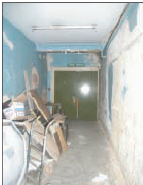
Plate 29 Room 26, hallway leading to the porch, looking south
