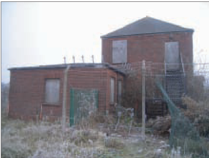
Plate 4 Western end of the building, looking east
