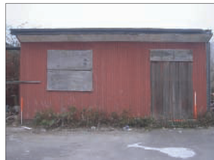
Plate 42 Temporary construction outbuilding, looking north-east
