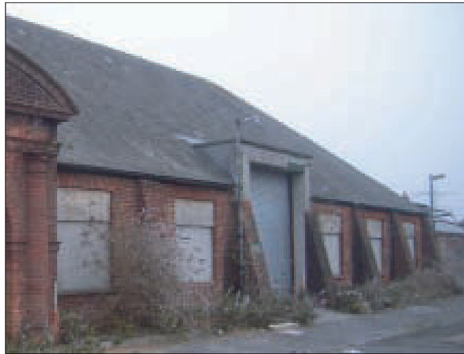
Plate 2 South elevation of the central block, looking north-east
