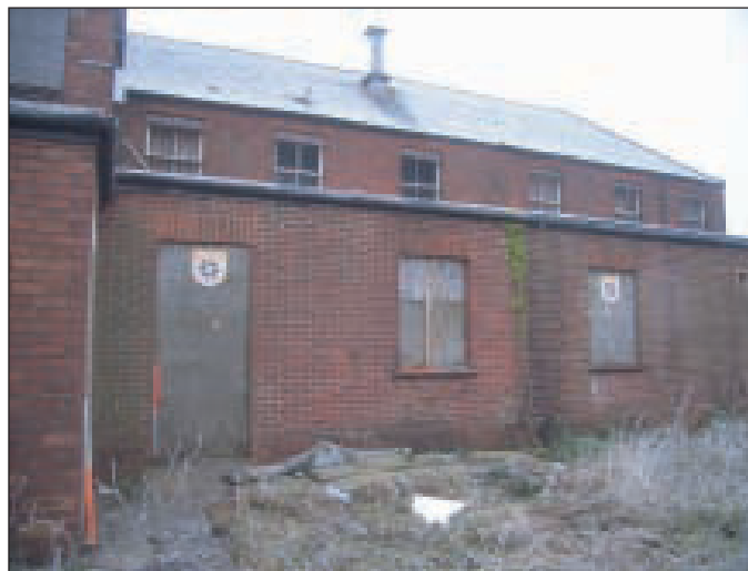
Plate 5 North (rear) elevation of west end of the building, looking south-west
