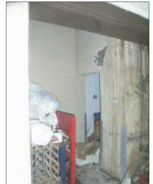
Plate 36 Room 5, looking north-west
