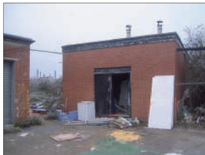
Plate 41 Brick built outbuilding, looking north-east
