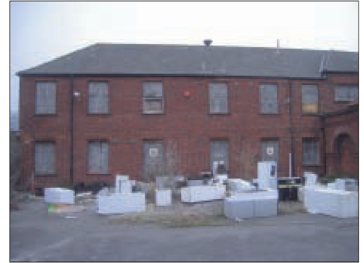
Plate 3 South elevation of the two storey block, looking north
