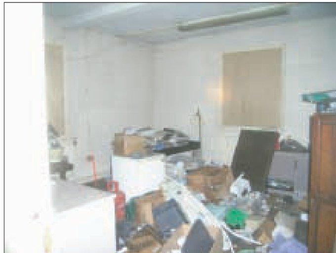
Plate 26 Room 23, looking north-west
