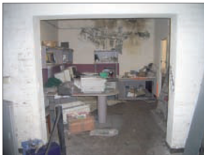
Plate 11 Room 3, looking east
