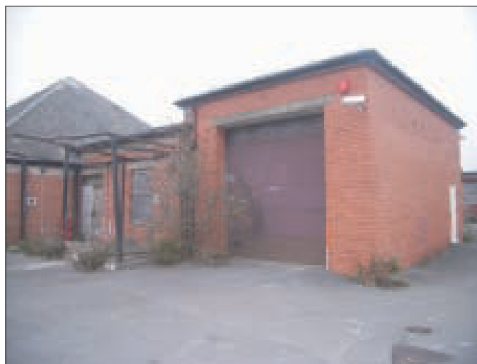
Plate 8 South and east elevations of the east end of the building, looking north-west
