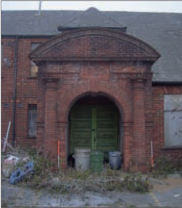
Plate 1 Front view of the brick porch, looking north
