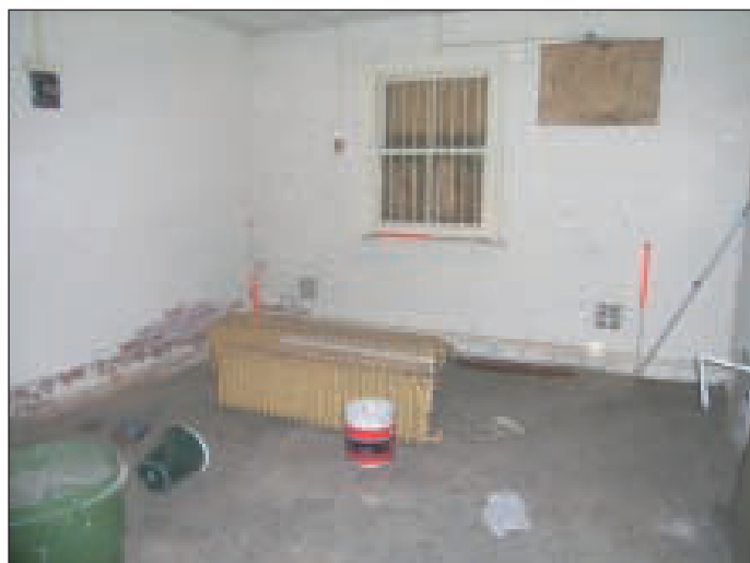
Plate 28 Room 25, looking north-west
