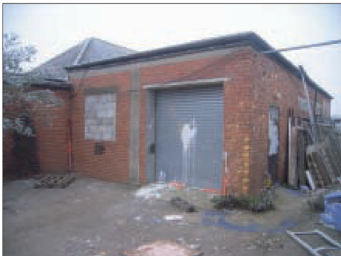
Plate 7 North and east elevations of the English garden wall bond block, looking south-west
