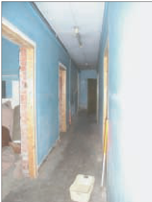
Plate 19 Ground floor corridor, Room 16, looking west
