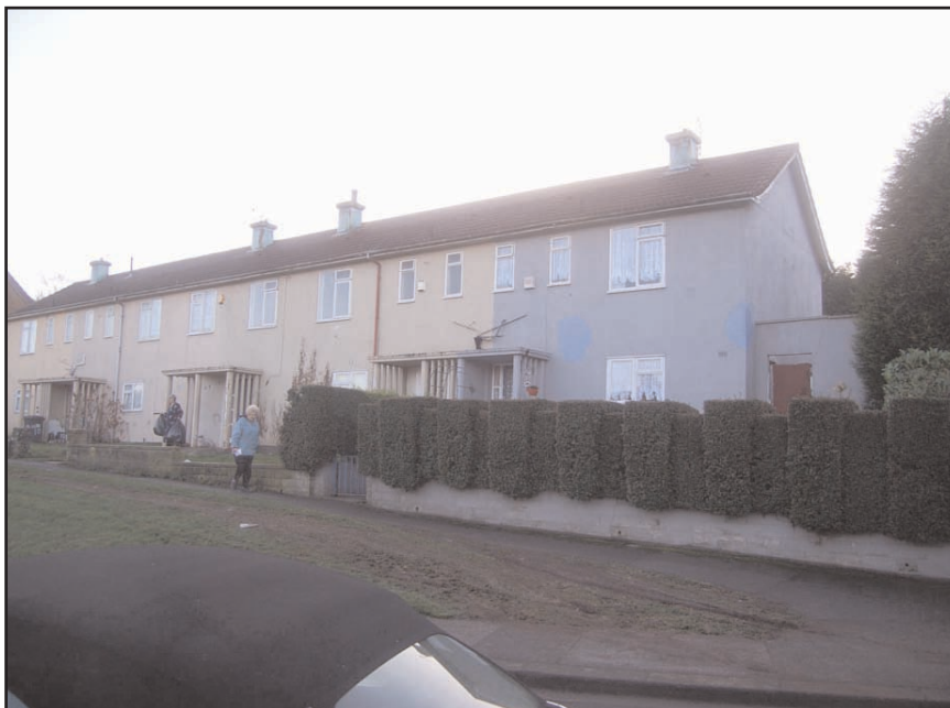
Plate 5 Frontages of Nos 6, 8, 10 & 12 Commonfield Road, looking ESE (Woolaway Type E)
