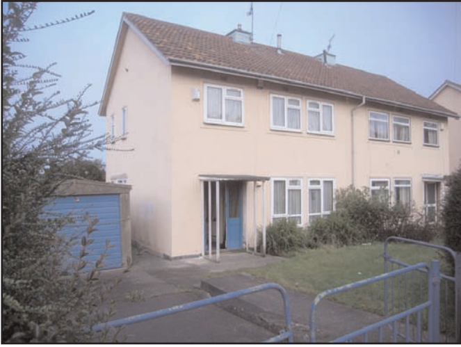
Plate 13 Detail of the frontage of Nos 17 & 19 Constable Road and the south- west facing elevation of No 17, looking N (Woolaway Type A)
