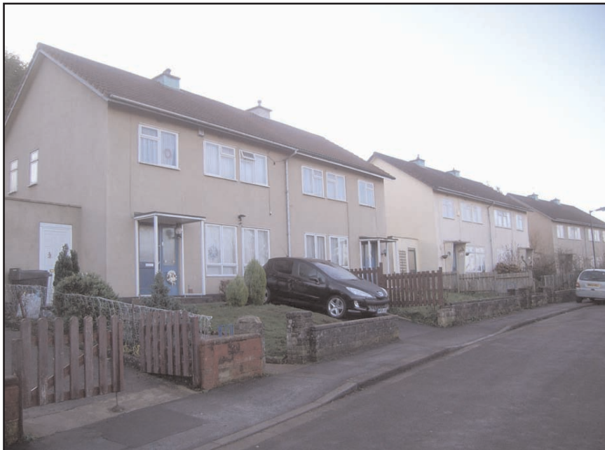
Plate 8 Frontages of Nos 11 – 16 Astry Close, looking SSW (Woolaway Type A)
