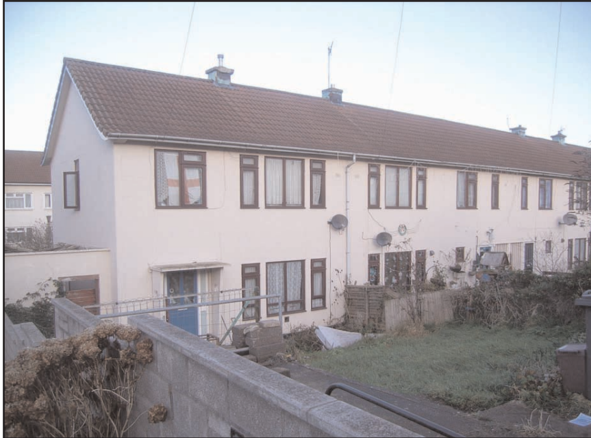
Plate 4 Oblique view of frontage of Nos 23, 25, 27 & 29 Capel Road, looking N (Woolaway Type D)
