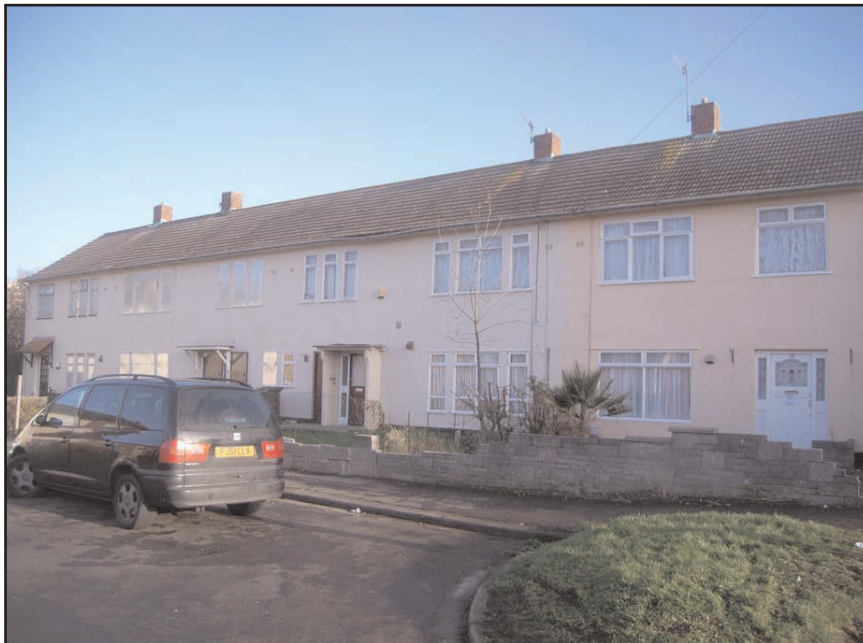
Plate 11 Frontages of Nos 11 – 14 Richeson Close, looking NE (Woolaway Type F)
