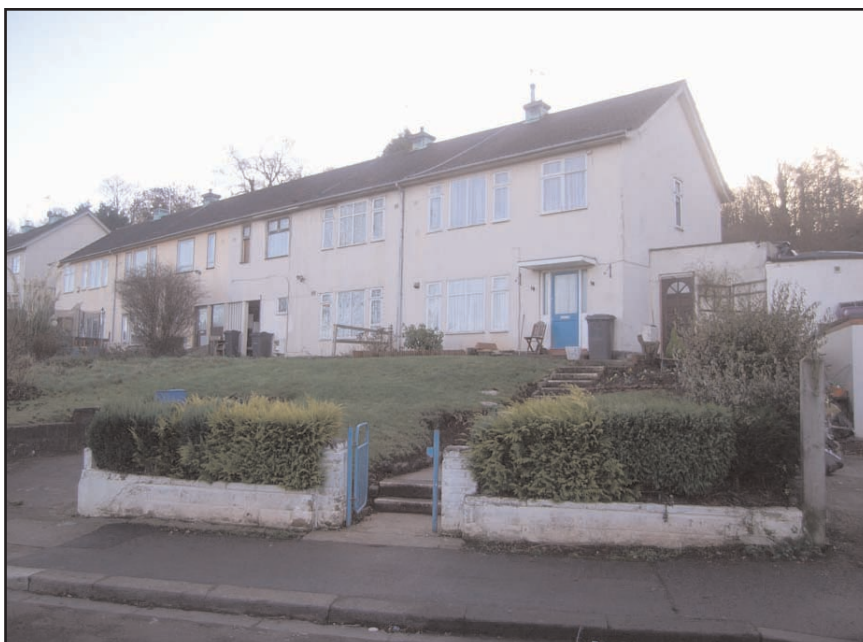
Plate 6 Frontage of Nos 1 - 4 Littlemead, looking E (Woolaway Type D)
