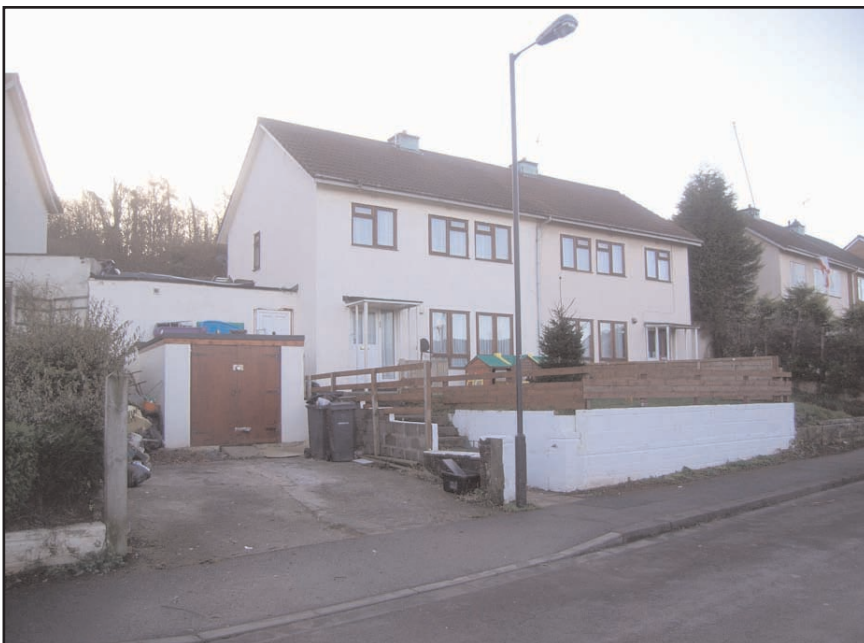
Plate 3 Frontage and north-east elevation of Nos 18 & 20 Oakhanger Drive, looking south (Woolaway Type C)
