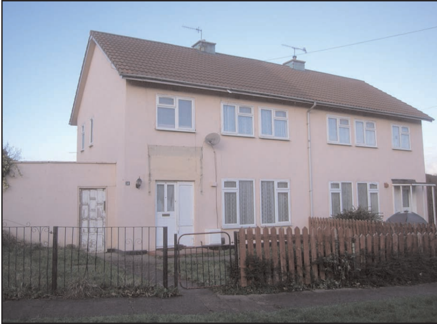
Plate 1 Detail of Nos 14 & 15 Knovill Close frontages, looking NW (Woolaway Type A)
