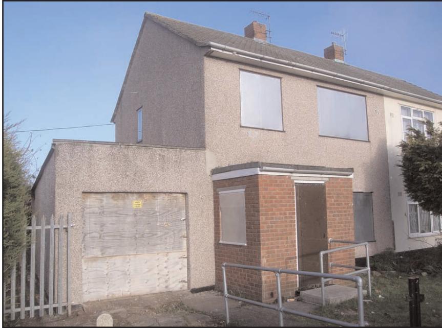
Plate 10 Detail of the frontage and south-west facing elevation of No 1 Monsdale Close, looking NE (Woolaway Type H)
