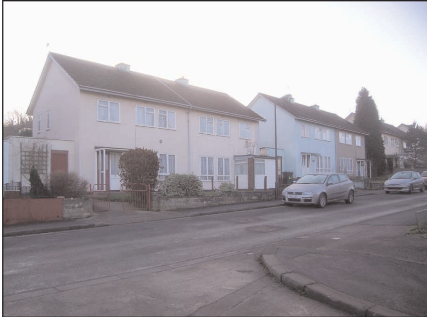
Plate 7 Frontages of Nos 3 – 6 Deans Mead, looking S (Woolaway Type A)
