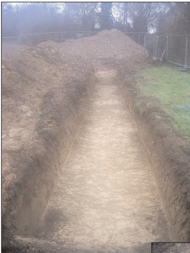
Plate 4 Trench 7, looking west
