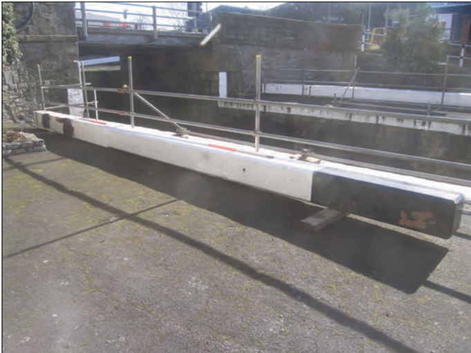
Plate 16 Lower lock north side balance beam, looking south-east
