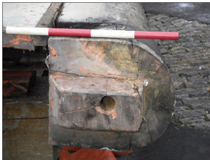
Plate 20 Top of the upper south gate, balance beam fixing, south side
