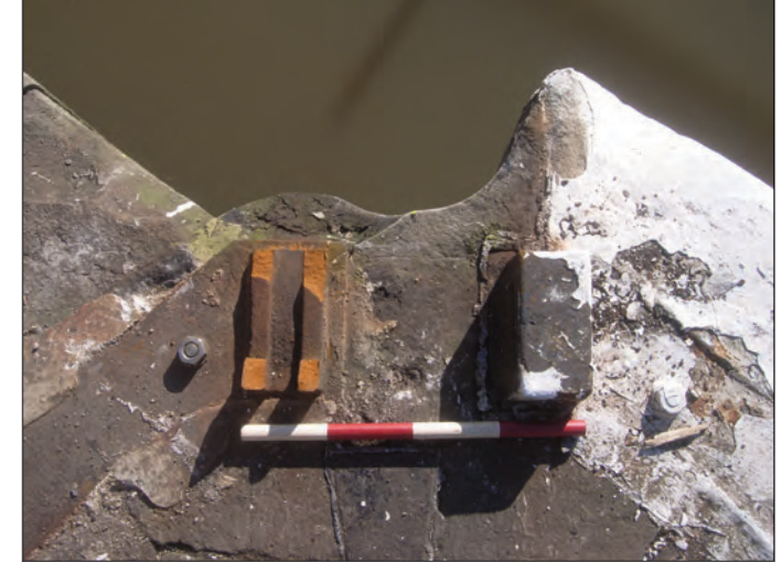
Plate 12 North side of lock, lower gates fixing brackets, looking south-east
