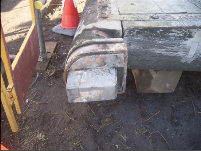
Plate 7 Lock-side fixing for the balance beam on the upper section of the lower north gate
