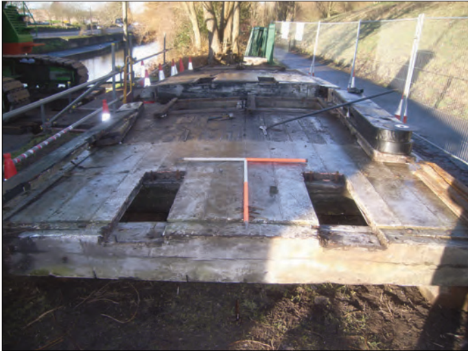
Plate 1 South gate of the lower lock gates, east face viewed from the top
