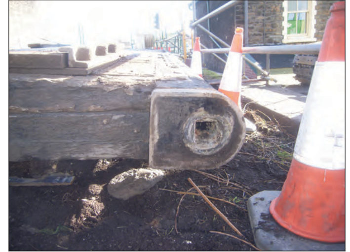
Plate 9 Base of the lower north gate pintle point
