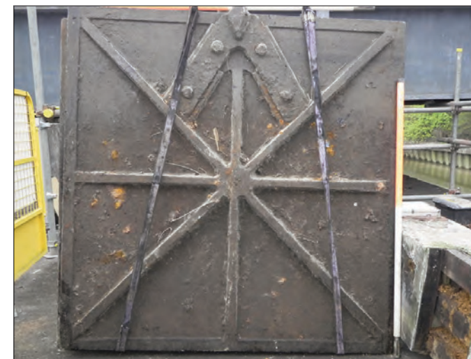
Plate 21 Sluice paddle of the upper gates
