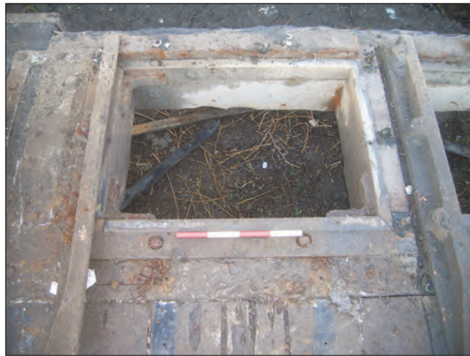
Plate 5 North sluice of the lower south gate, with alterations made to three of the corners, east face
