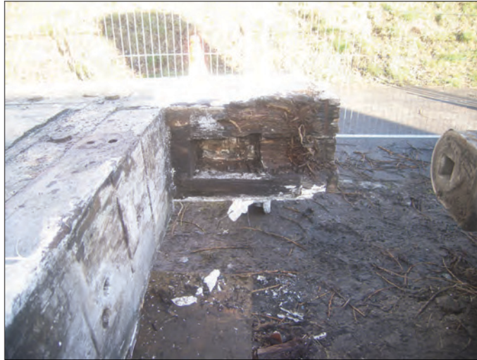
Plate 8 Centre of the lock fixing for the balance beam on the upper section of the lower north gate
