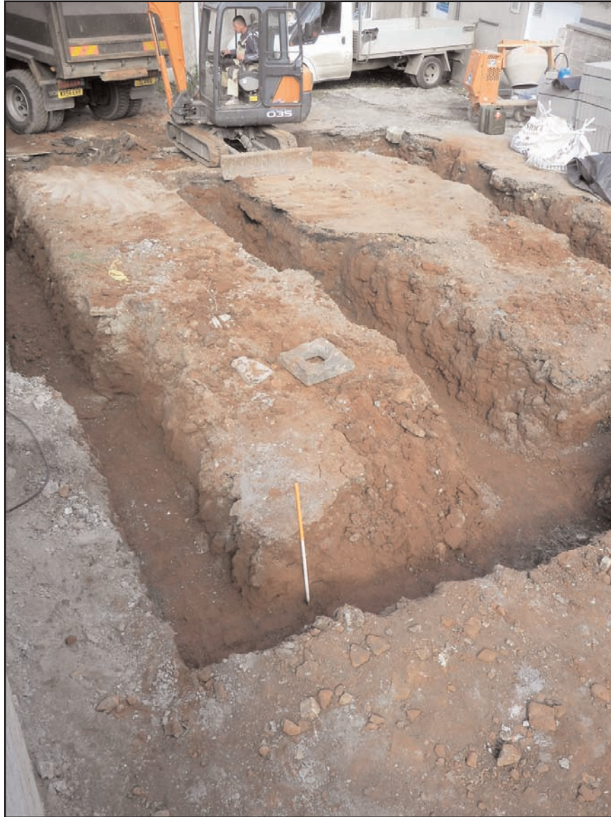
Plate 4 General view of the footings, nearing completion, looking north-east, scale 0.5m
