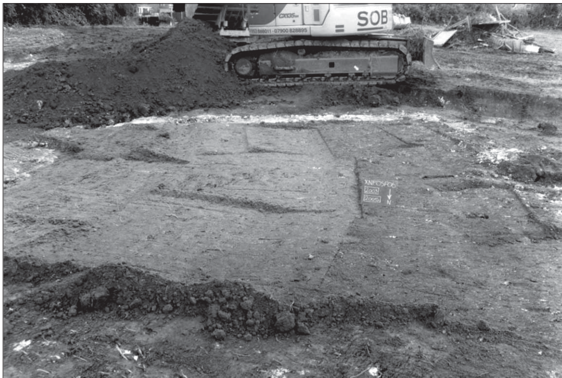
Plate 12: Building 5 - chalk foundations cutting through subsoil 2001, from the north
