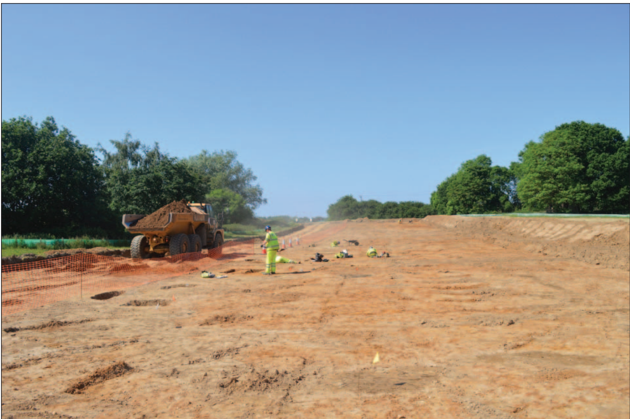
Plate 18: Area 13 under excavation, looking north
