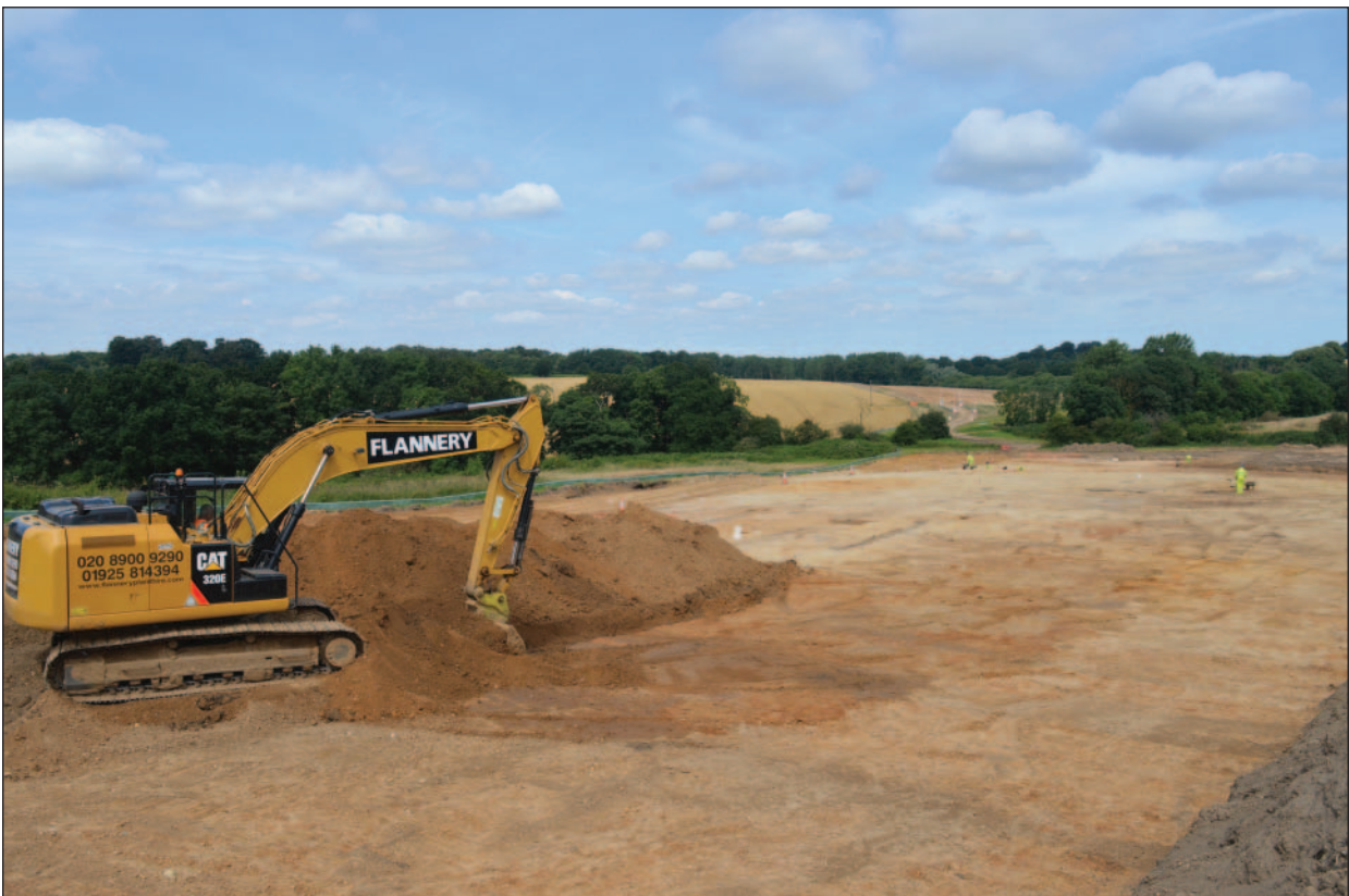
Plate 16: Area 12 under excavation, looking north-north-west
