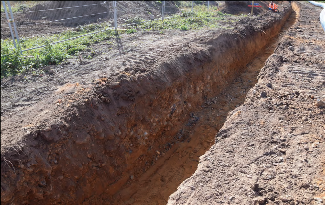
Plate 1: Pipe trench, chainage 1320, looking south-west
