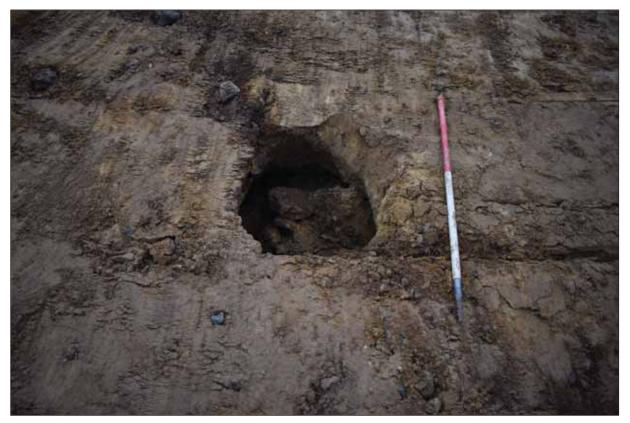
Plate 4: Active/new sinkhole opening during machining of the site
