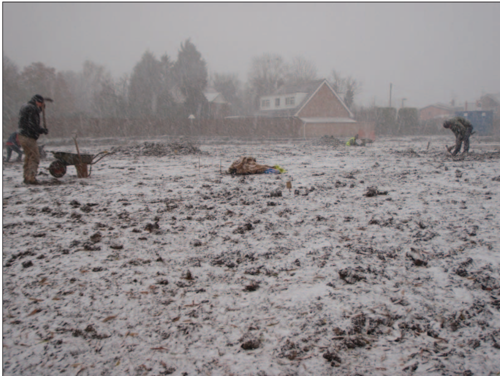
Plate 2: Working in poor conditions, looking south-east
