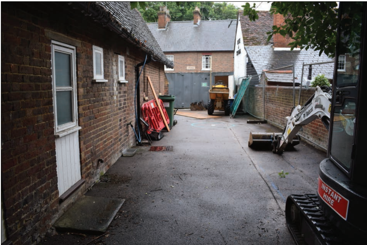
Plate 1: General view of excavation, viewed from the north-west
