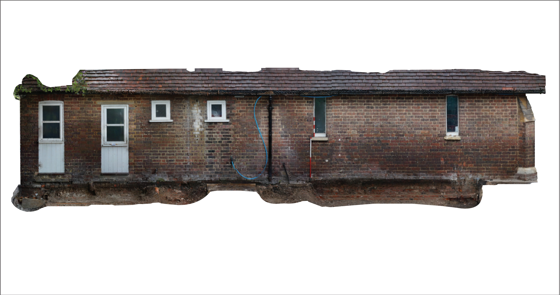
Figure 12: Photogrammetric image of the south-west elevation of the school
