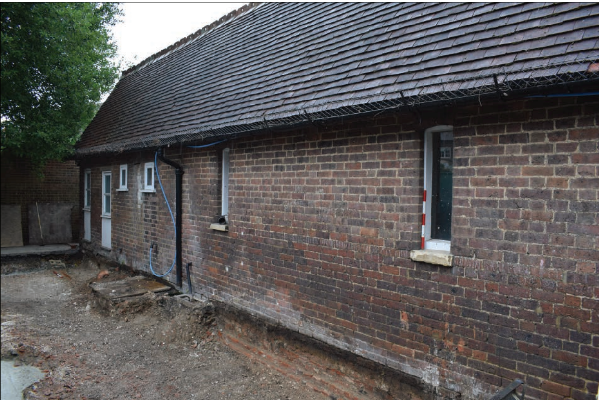
Plate 26: Oblique view of the south-west elevation of the school
