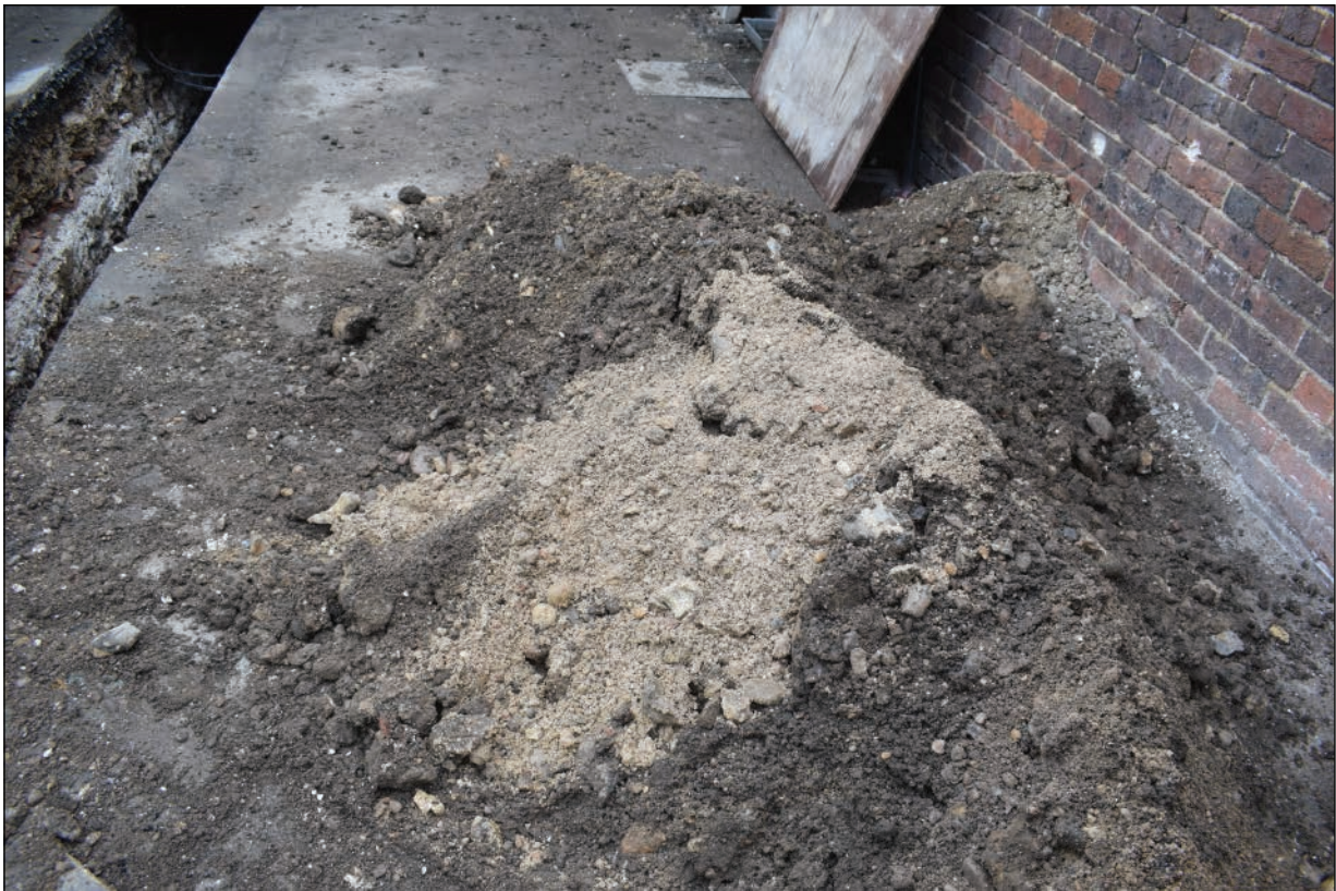
Plate 22: Detail of lime mortar 127
