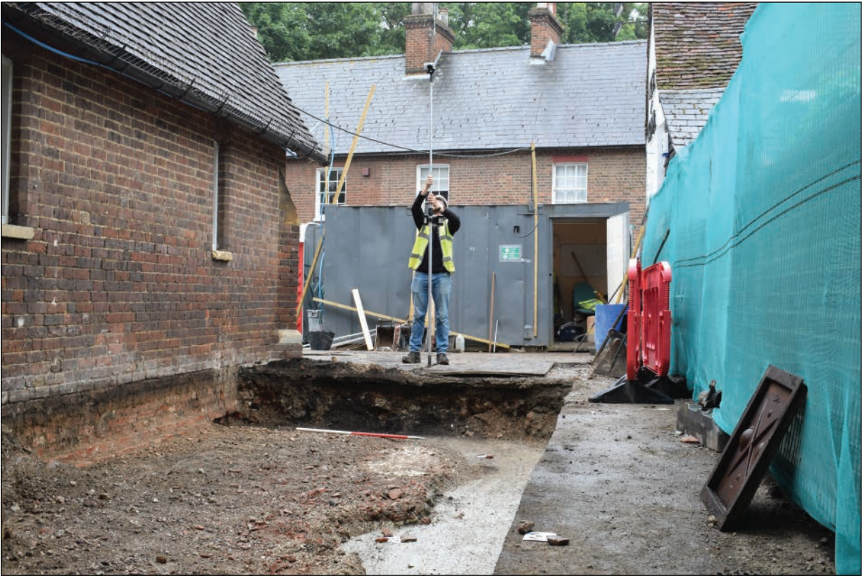
Plate 27: Photogrammetric recording of the excavation area
