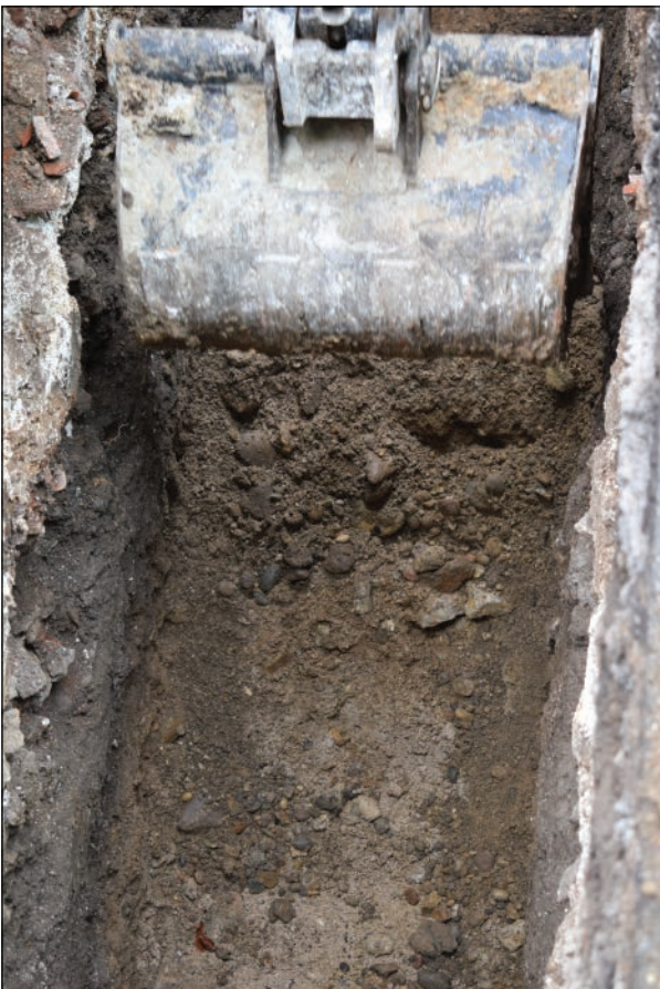
Plate 20: Lower levels of the trench, showing mortar layers 110 and 127
