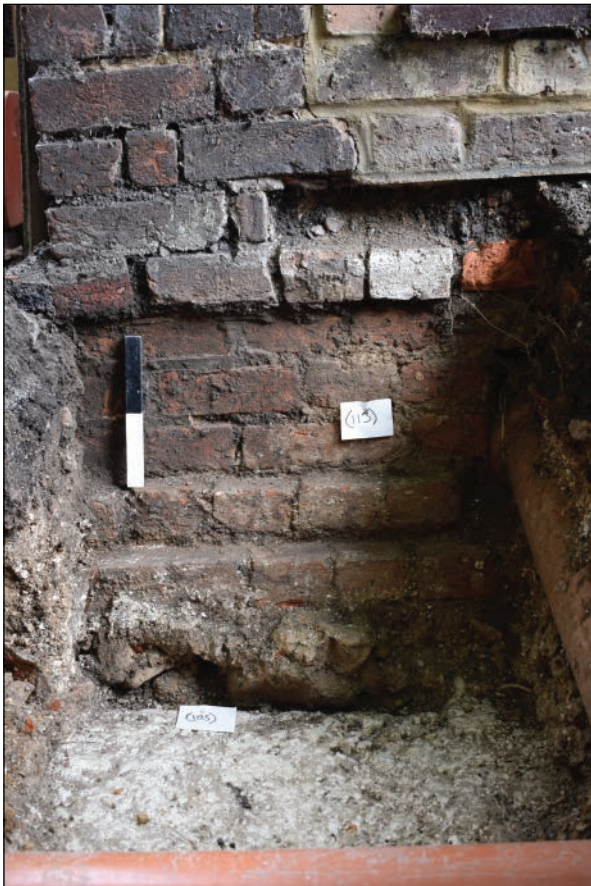
Plate 4: School foundation truncating chalk raft 105, viewed from the south-west
