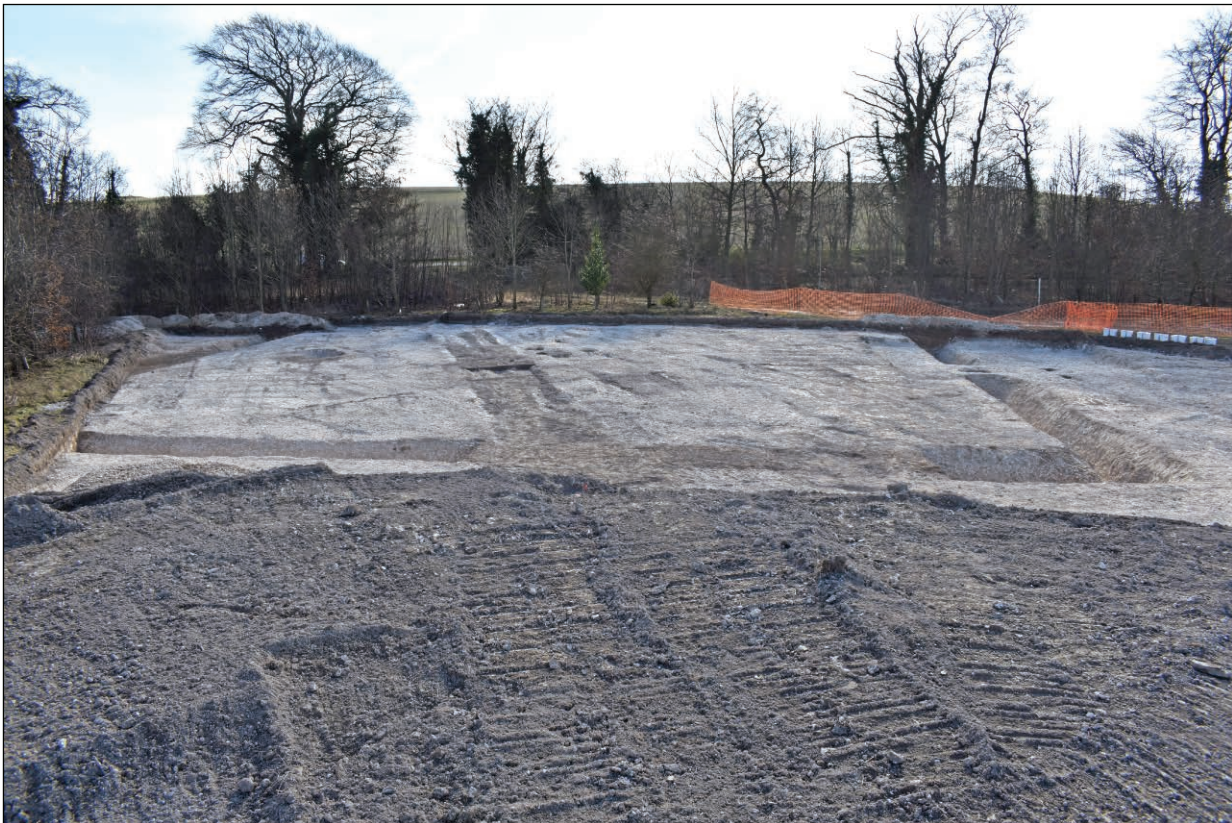
Plate 3: Post-excavation shot of the site from the north
