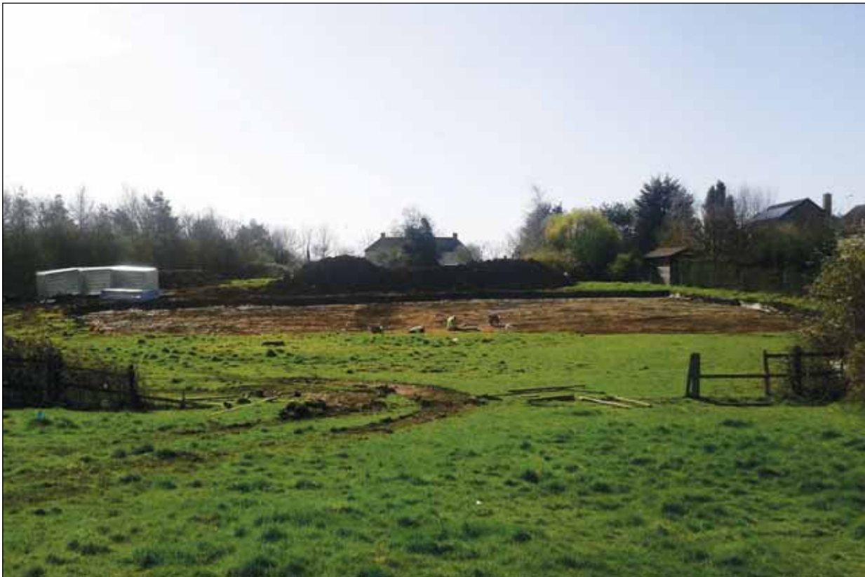
Plate 2: View of site, looking south (showing Area 1 during excavation)
