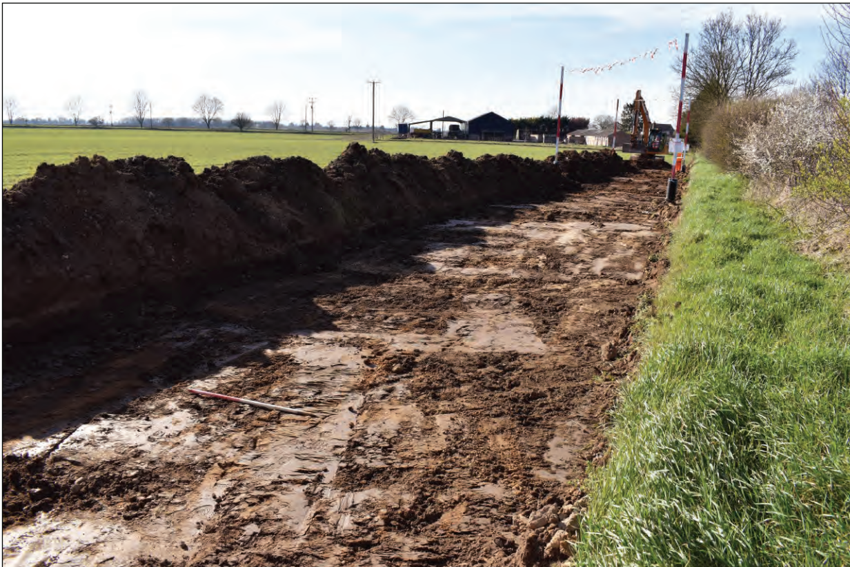
Plate 4: North-west to south-east part of strip, north-west end, looking west
