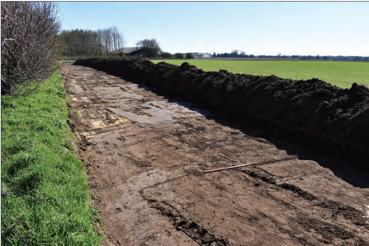
Plate 2: North-west to south-east part of strip, south-east end, looking south
