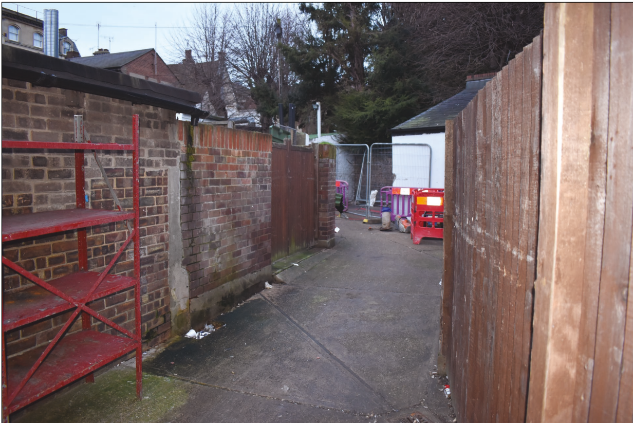
Plate 2: Pre-excitation (Trench 2), looking north along pipe route
