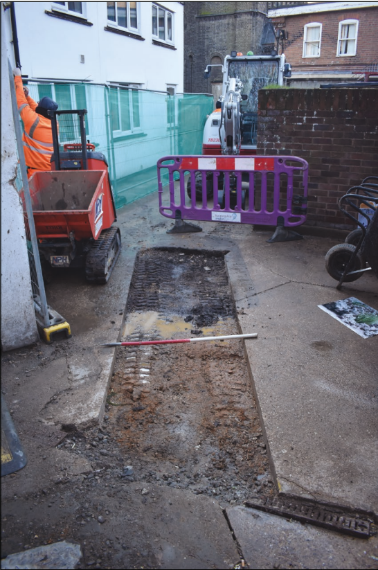
Plate 3: Pre-excavation (Trench 2), looking south-east along pipe route
