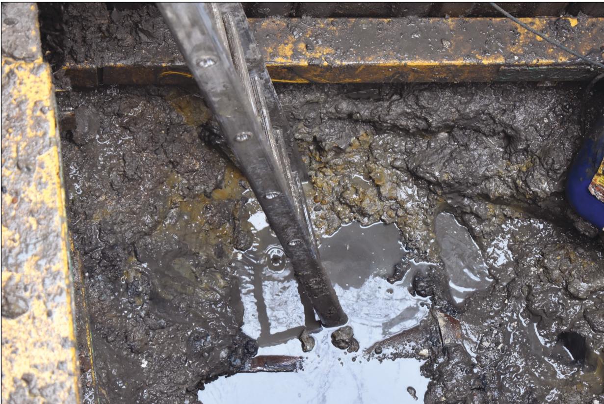
Plate 4: Working shot (Trench 1) showing geology and pipe
