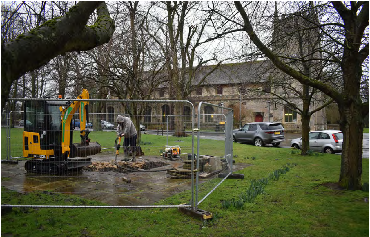
Plate 1: Drilling work in progress, from the northwest
