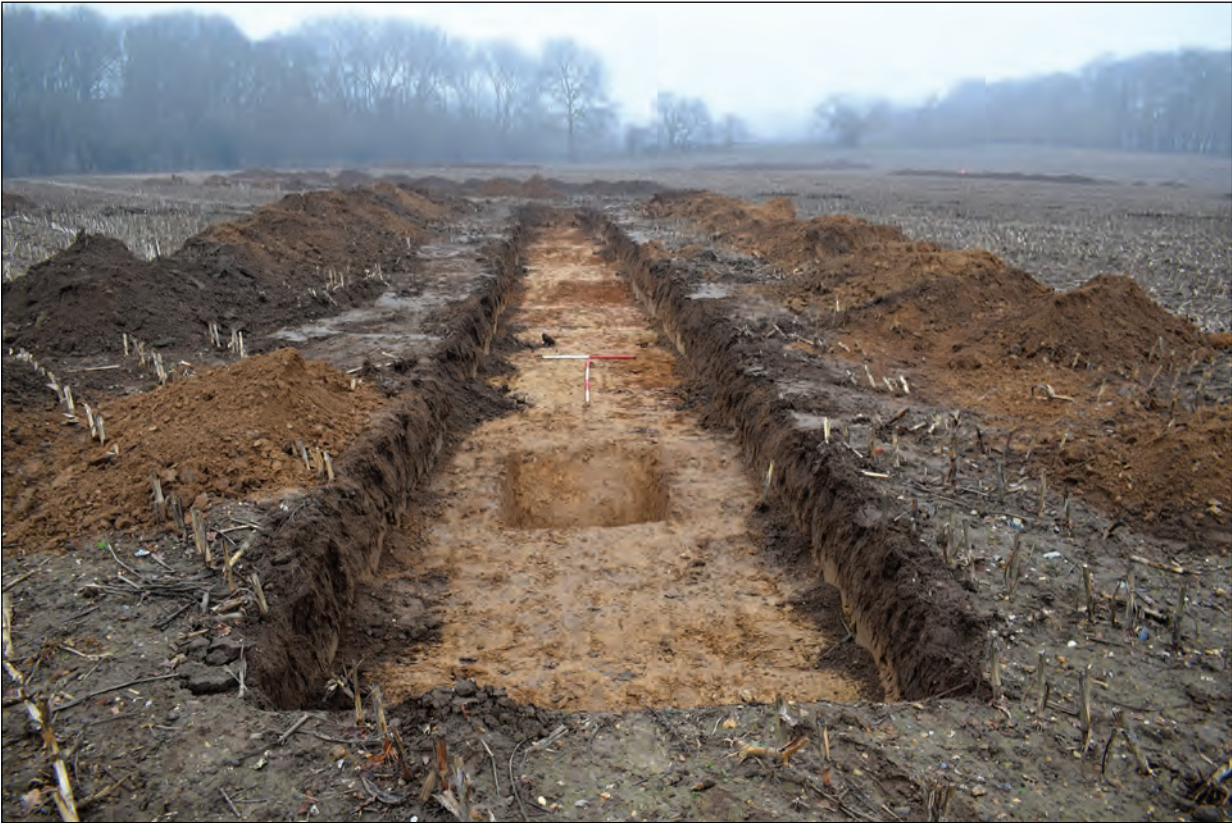
Plate 11: Trench 8, from the north
