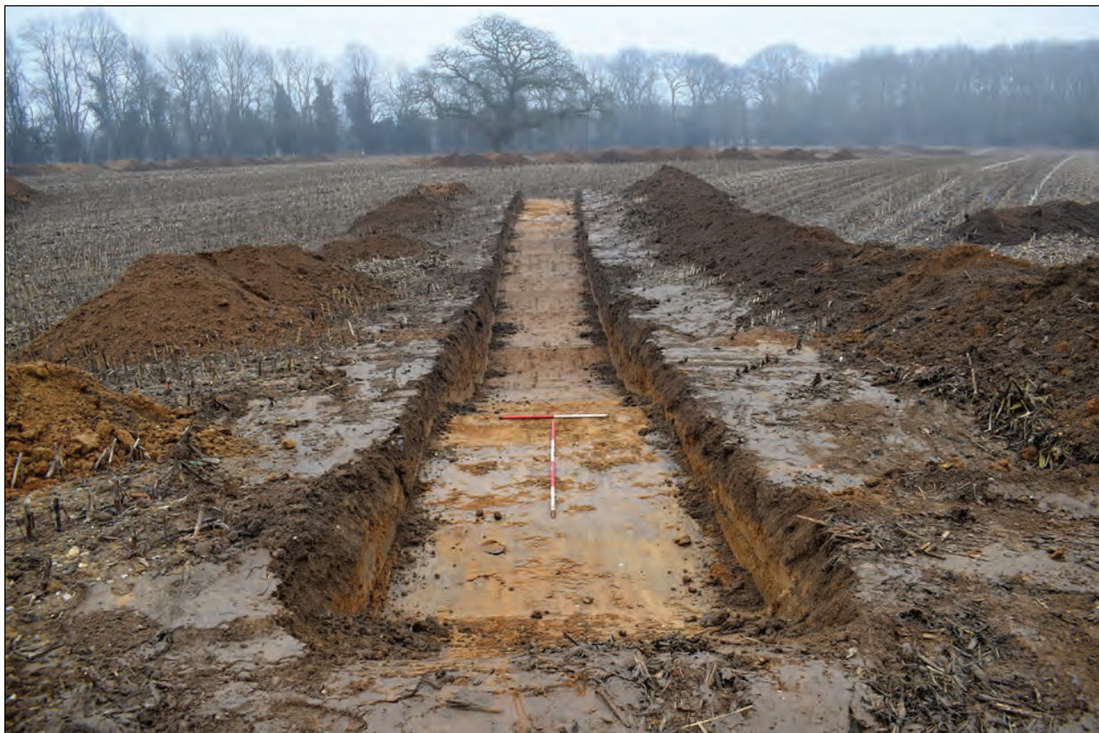
Plate 14: Trench 10, from the north-west
